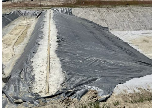
An impervious liner in the forebay and inlet batter or an inground SRP constructed in glacial till soils.
