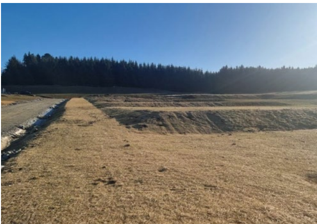
Use a dense hay mulch layer, watered in, to provide superior ground coverage, anchoring, and moisture retention compared to straw or lightweight hydromulches, particularly on erosion prone soils.
