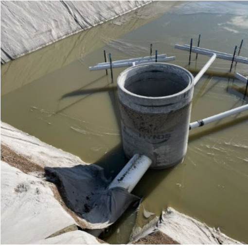
An SRP outlet batter constructed above ground in glacial tills has failed due to backward erosion along the outlet pipe.
