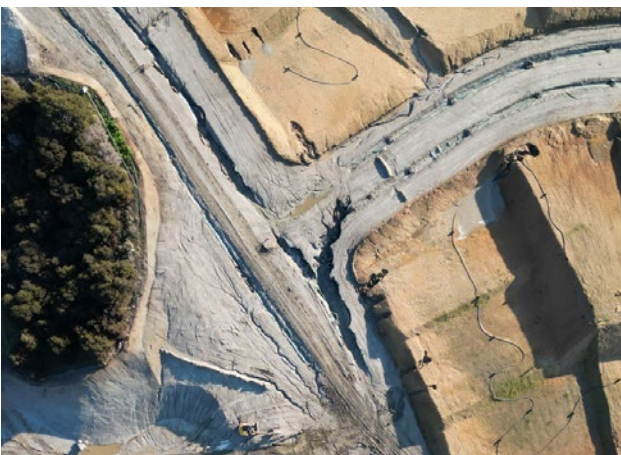
Significant damage to a dirty water diversion channel constructed in glacial till soils.
