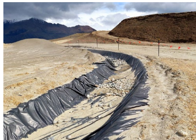
More conservative, flatter grade dirty water diversion channel with step downs protected with rip rap.
