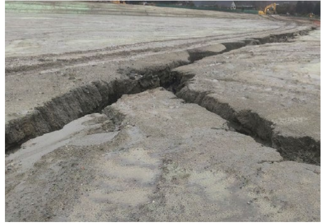
Significant rilling through glacial till on a large site which has turned sheet flow in to highly erosive concentrated flow
