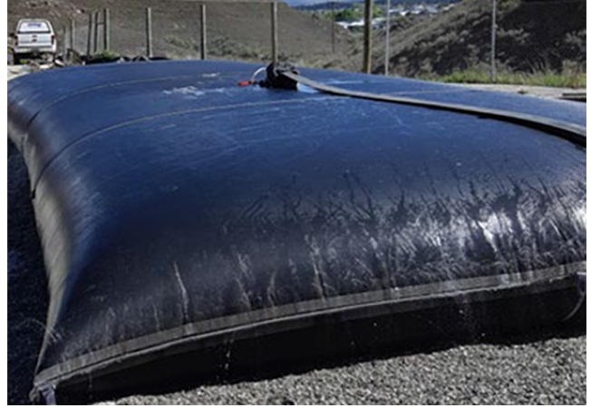
Dewatering bags as a method to treat water before returning it back to a waterbody.
