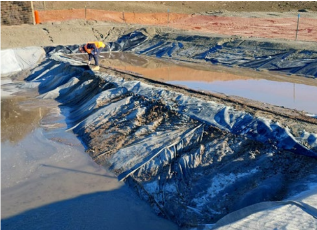
An SRP inlet batter lined with geotextile material getting significantly eroded in glacial till soils.
