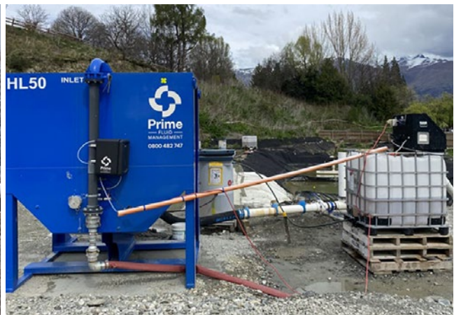
Water treatment system / settlement tank as part of the treatment train
