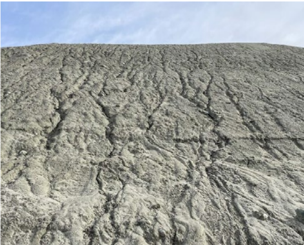
Rilling of a stockpile.
