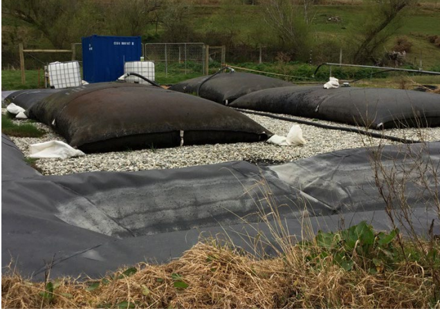
Dewatering bags as a method to treat water before returning it back to a waterbody.
