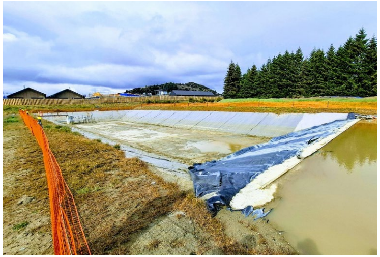
An SRP constructed in ground in glacial till soils reduces risk of batter failure.
