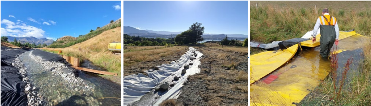
Examples of temporary diversion channels in Otago
