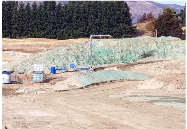
Polymer – long-term stockpile option with polymered stockpile with the surrounding area hydroseeded. Polymers form chemical or physical bonds with soil/plastic particles, creating a cohesive mass or a protective layer.
