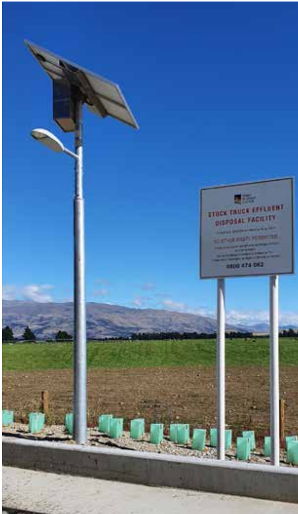
The new stock truck effluent disposal site at Tarras is now operational.
