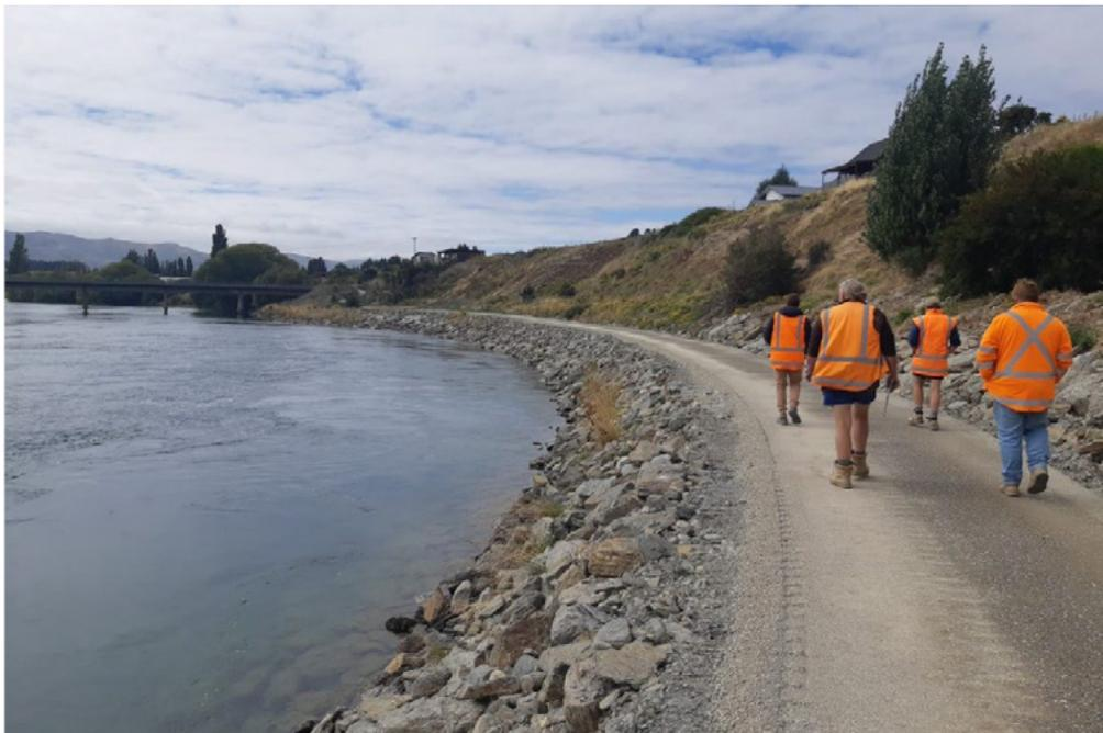
Figure 2 River channel asset, Albert Town (Clutha River/ Mata-Au) Rock Buttress flood repair works completed in February 2021.”
