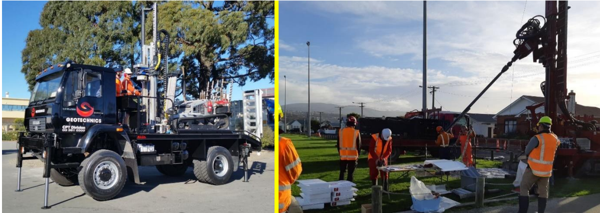
Figure 2: Examples of CPT testing equipment (left), and a drilling rig working on a similar geotechnical investigation programme in Dunedin (right).
