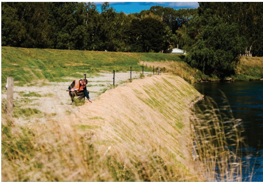
➡ New flood banks - Stirling, South Otago
