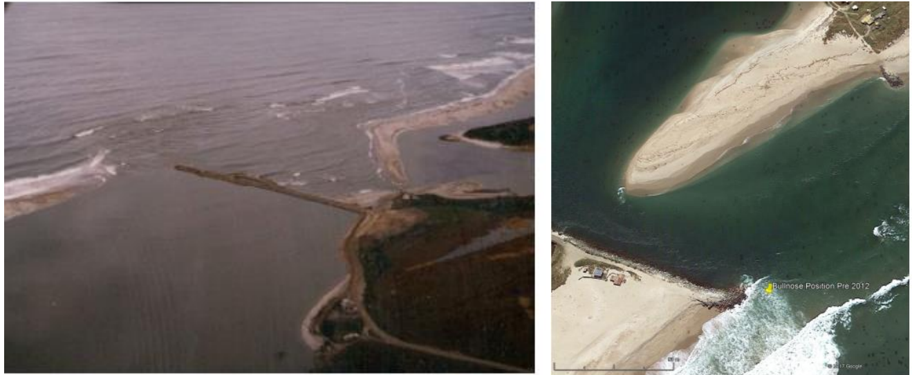
Figure 2.7: South training wall at the Koau River mouth. Photo A (left) - Under construction in May 1983; Photo B (right) – In 2016 from google earth imagery. Note the end of the northern wall can also be seen (Source: Bloor, 2017).
