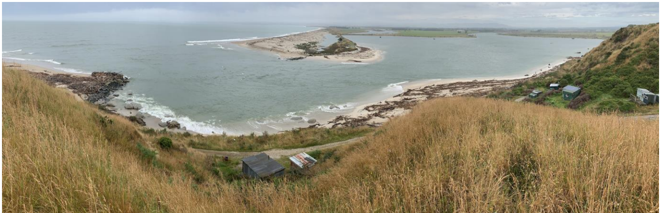
Figure 2.10: Matau River mouth looking south from Summer Hill showing the southern training line and the small northern rock groyne (Supplied by ORC, 2020).
