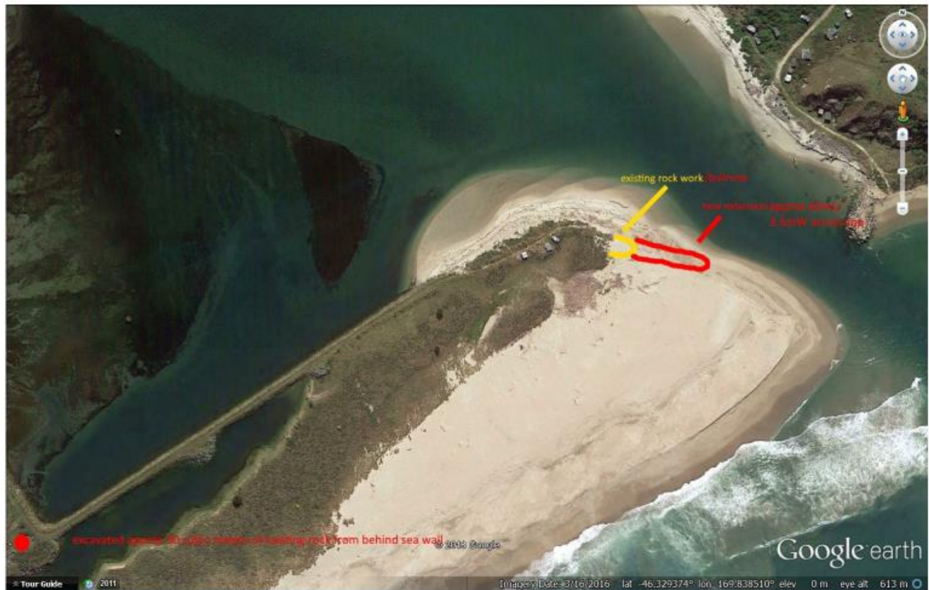
Figure 2.11: Matau River Mouth extensions of the southern training line in 1993 (yellow), and 2018 (red) (Source: GeoSolve, 2018).
