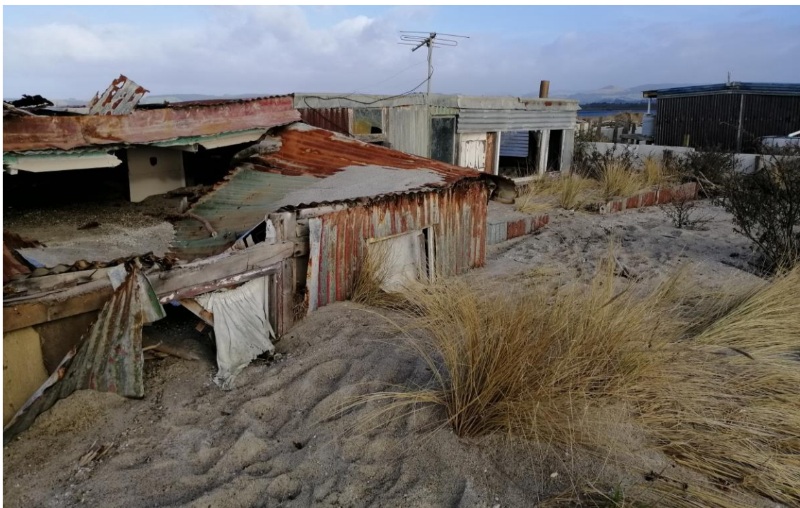
Figure 2.14: Evidence of wave overtopping south of the Koau Mouth southern training wall (Jacobs, 2020).
