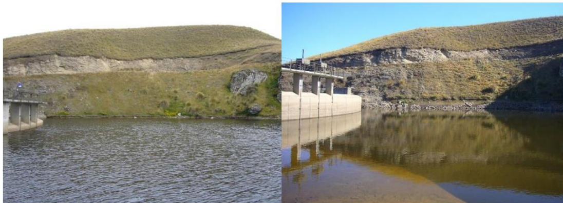
Figure 10: Lake Onslow dam at high lake levels (left) and with lake level 2-2.5 m below the crest. (Source: Further information)
