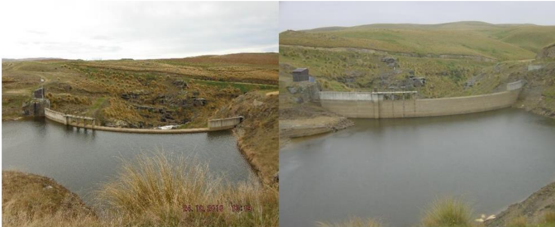
Figure 9: Lake Onslow dam at high lake levels (left) and with lake level 4.350 m below the crest. (Source: Further information)
