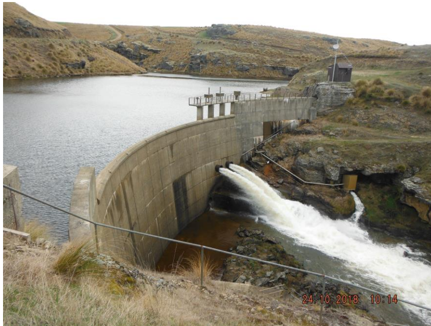
Figure 12: Lake Onslow dam with discharge into the Teviot River (Source: Further information)
