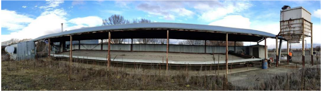
Figure 2: Oat processing facility
