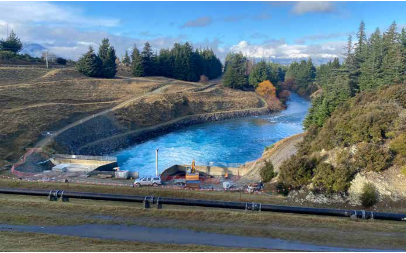
Figure 34 Hawea Control Dam
