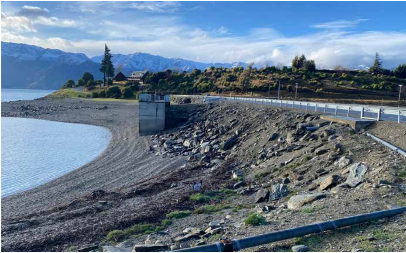
Figure 33 Hawea Control Dam
