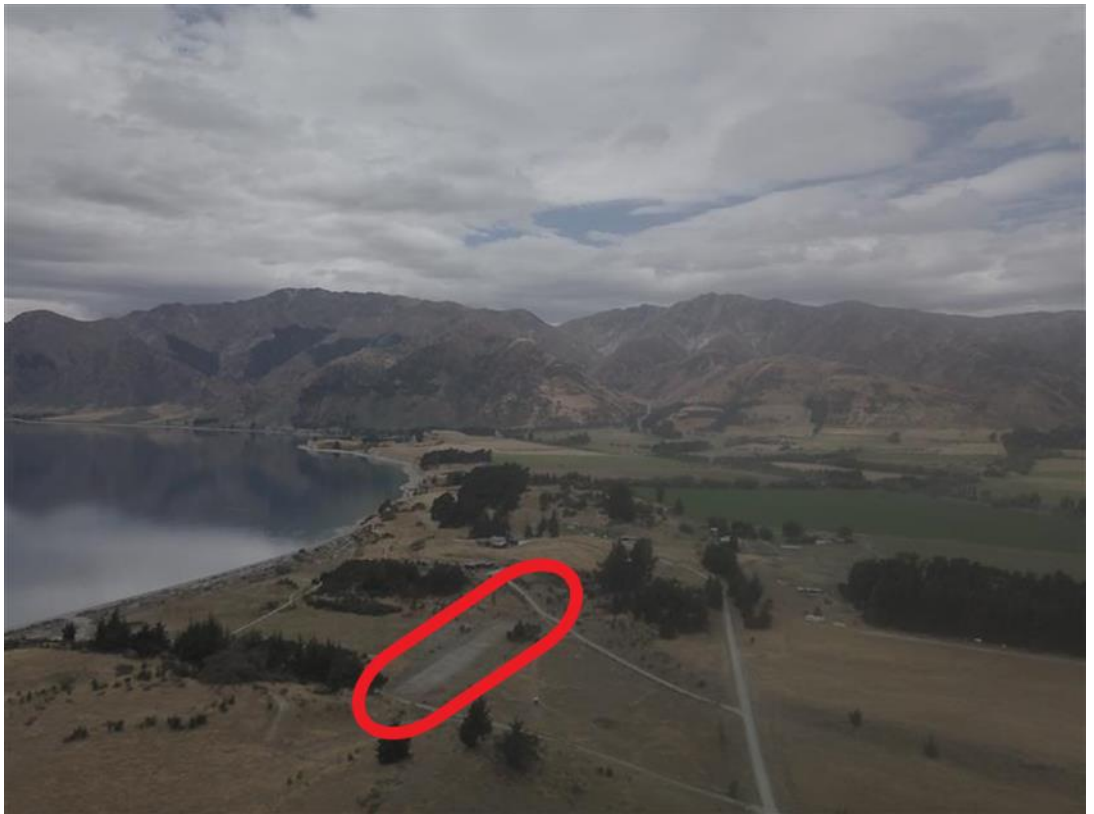
Figure 4: The Gladstone Gap Stopbank and Spillway
