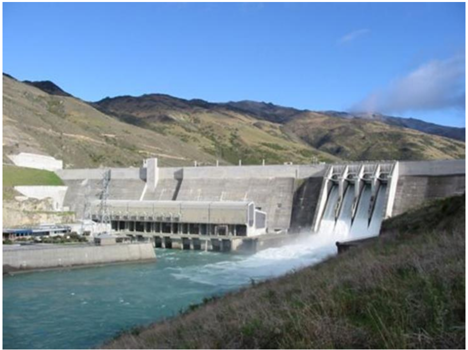
Figure 5: The Clyde Dam
