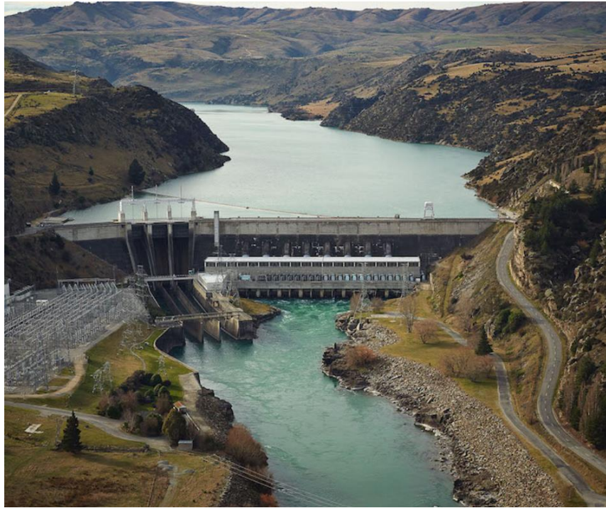
Figure 7: The Roxburgh Dam
