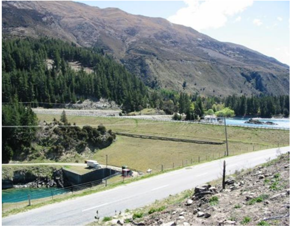
Figure 3: The Hāwea Dam
