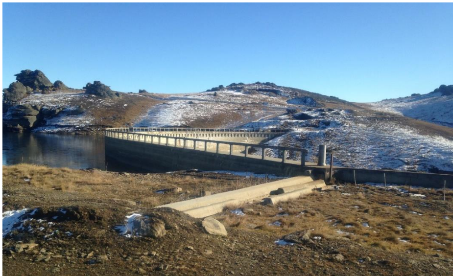
Photo Nine: View of Poolburn Dam – Concrete Arch Dam and Overflow Spillway on RHS of Dam
