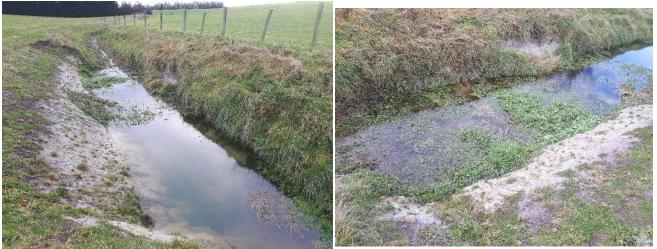
Another sediment trap that is now due for cleaning as it caught a lot of sediment during the February floods as they blew out the weed in places that was holding the sediment in the bed. Plant growth in a sediment trap seems to increase its efficiency at catching fine sediment as it slows down the water velocity and binds up the sediment in the base of the sediment trap.
