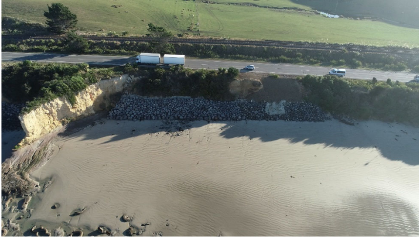
Figure 2: Coastal Protection Katiki Beach
