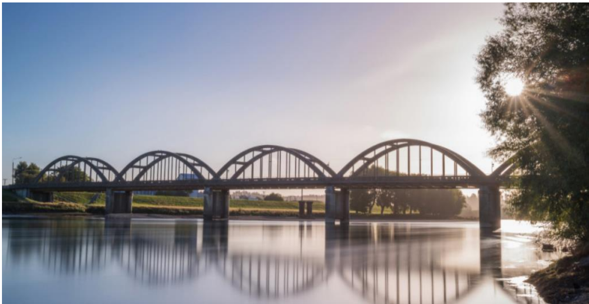
Image 1. The Balclutha bridge - One of New Zealand's most distinctive bridges links the two parts of the town. Built in the 1930s, the six-span arched concrete bridge has a Historic Places Grade 1 listing.
