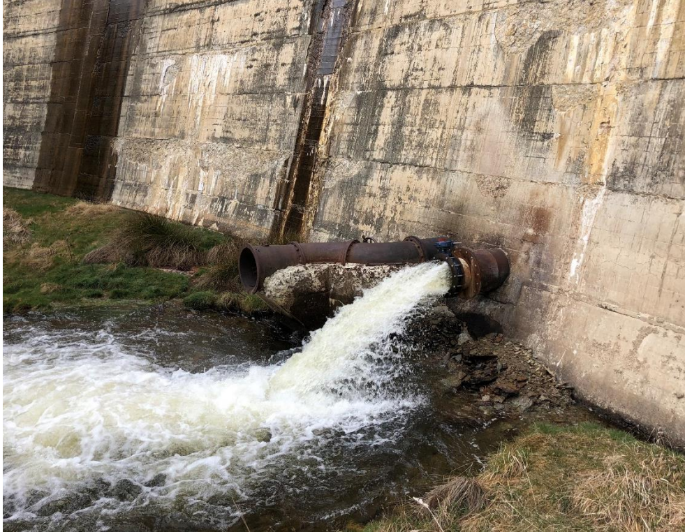
Photo Eleven: View of Poolburn Dam – Outlet Conduits (x2)
