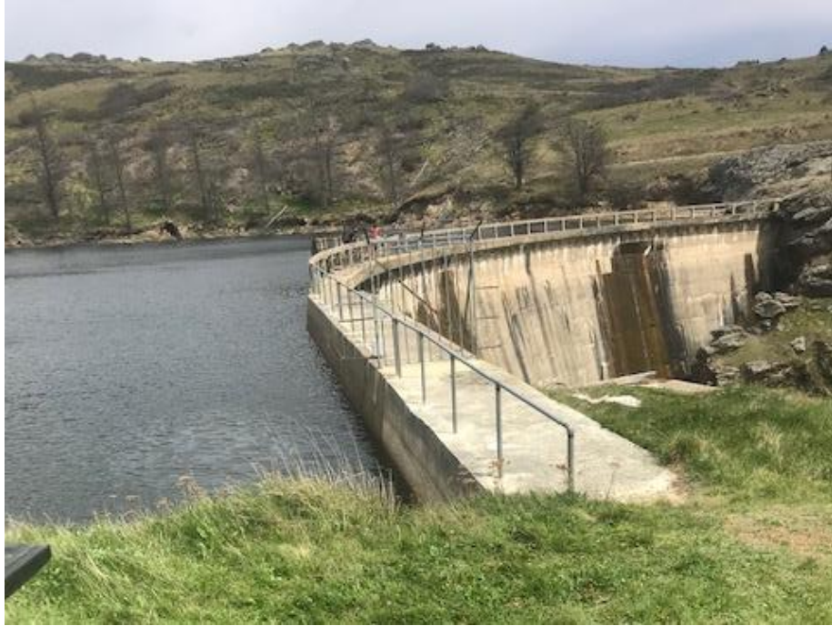
Photo One: View of Concrete Arch Dam
