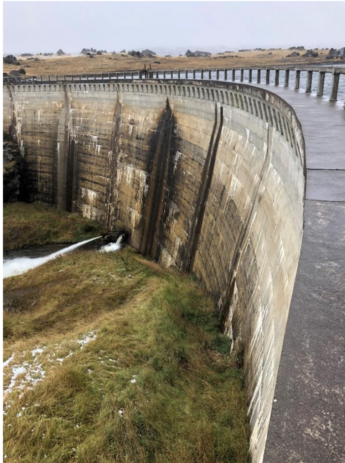
Photo Ten: View of Poolburn Dam – Concrete Arch Dam
