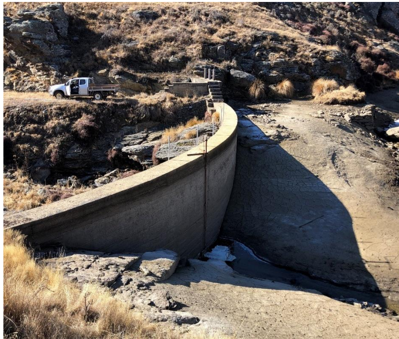
Photo Five: View of Upper Bonanza Weir – Concrete Arch Dam
