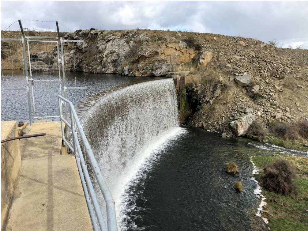
Photo Eight: View of Poolburn Weir – Concrete Arch Dam
