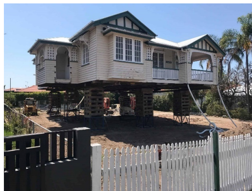
Figure 2.1: A house that is being raised [6].
