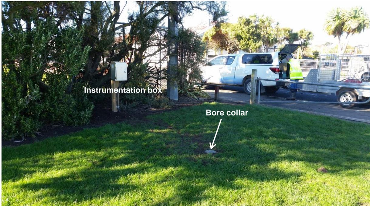
Figure 17. Typical example of an ORC bore installation, with bore collar and instrumentation box, at the Culling Park site.
