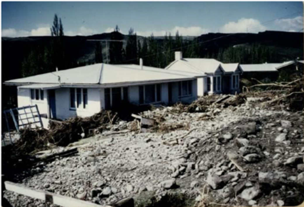
Figure 6: Direct impact of a debris flow at Reservoir Creek, 1978, showing extensive debris deposition, and direct impact to dwellings adjacent to the stream channel.
