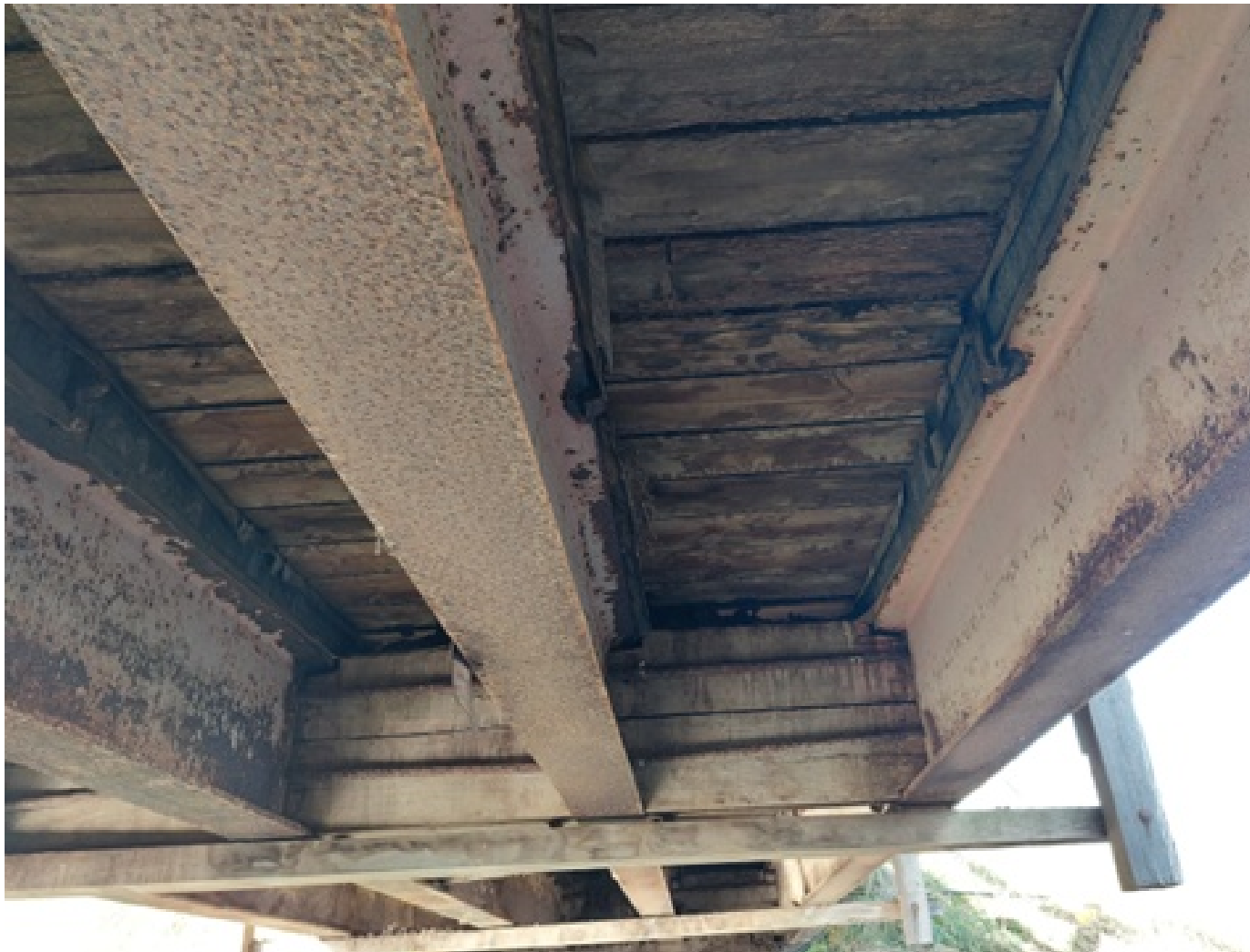
Figure 3: Underside of bridge 2 indicating significant corrosion of beams
