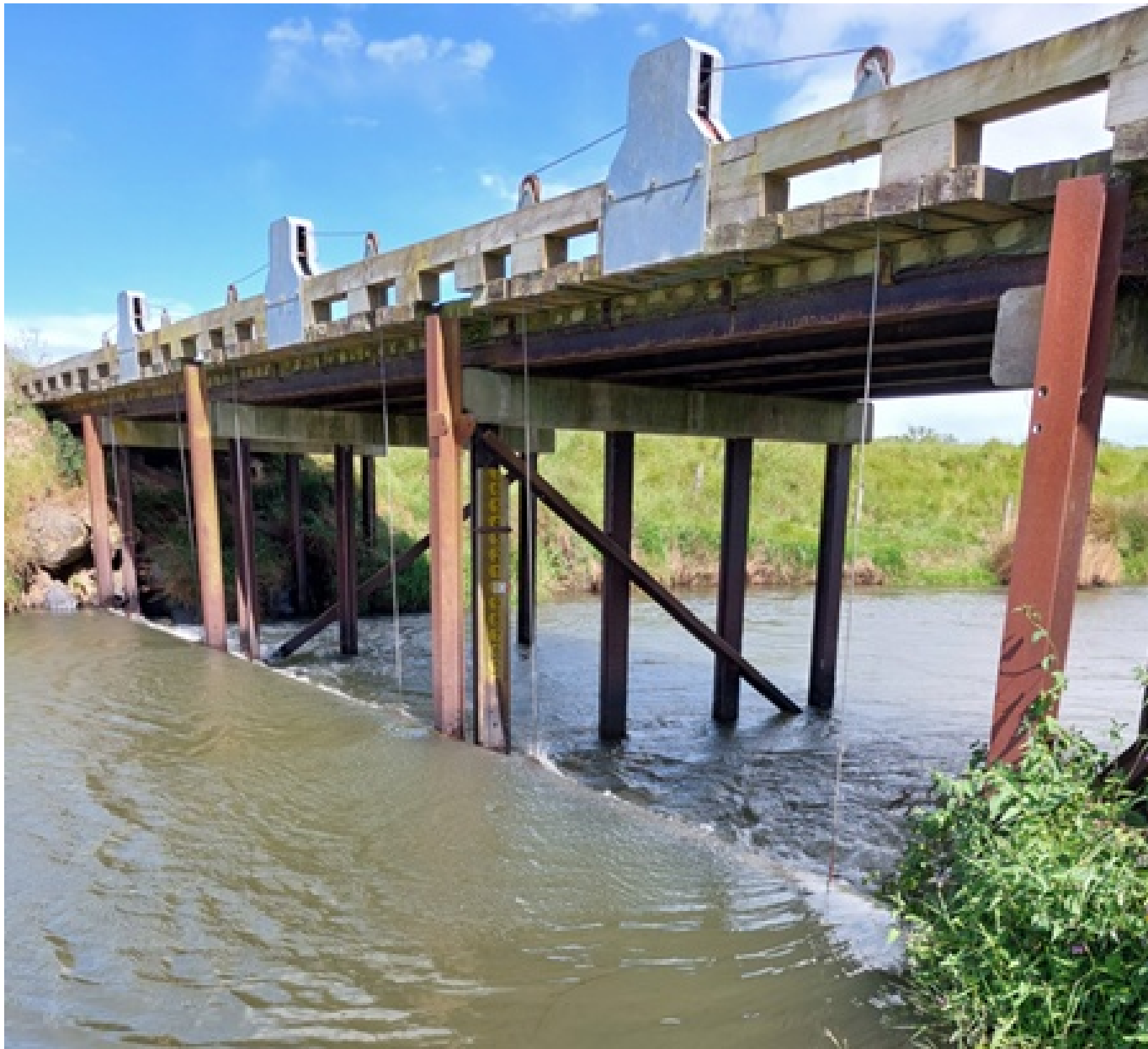
Figure 5: Drain 222 with sills in place.
