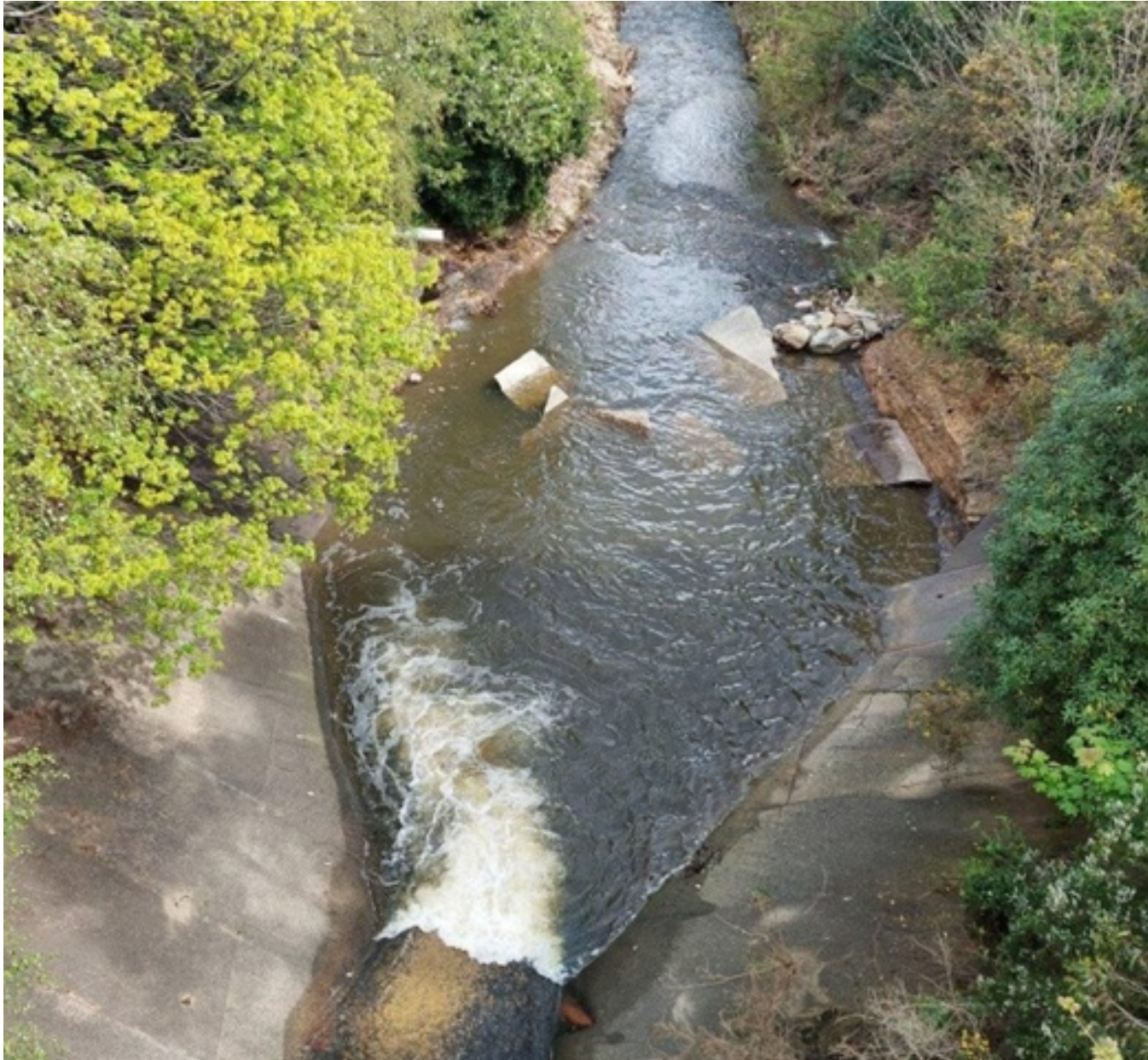
Figure 7: Kaikorai Stilling Basin indicating damage to concrete lining.
