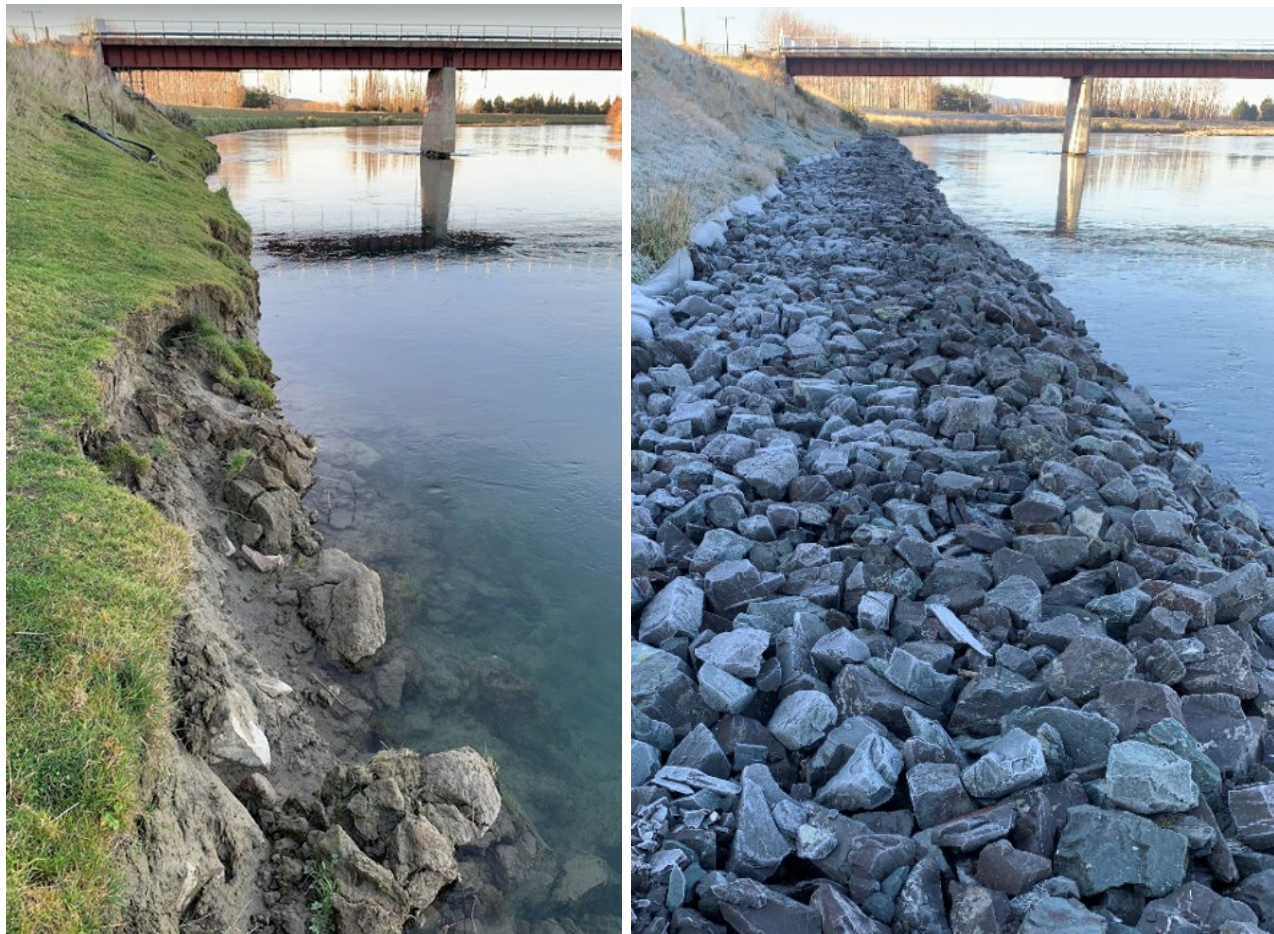
Figure 6: Riverbank Road floodbank at bridge near Stirling (LC21), before(left) and after (right) reshaping and vegetation stabilisation.
