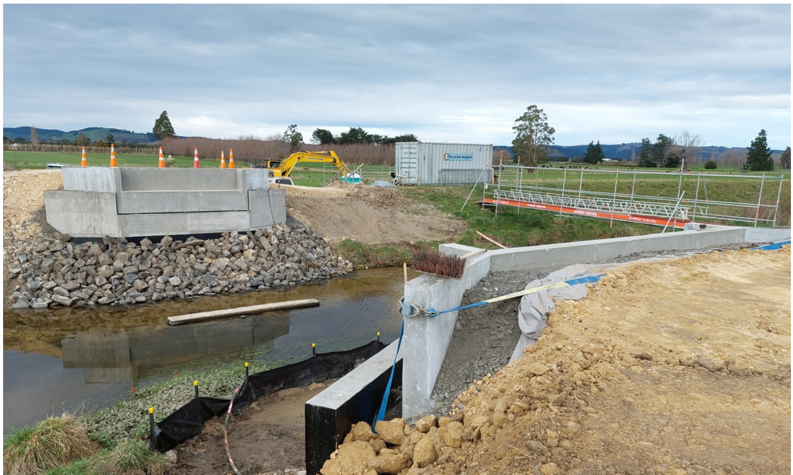
Figure 3: Bridge 11 replacement underway at Contour Channel (18 July 2023).
