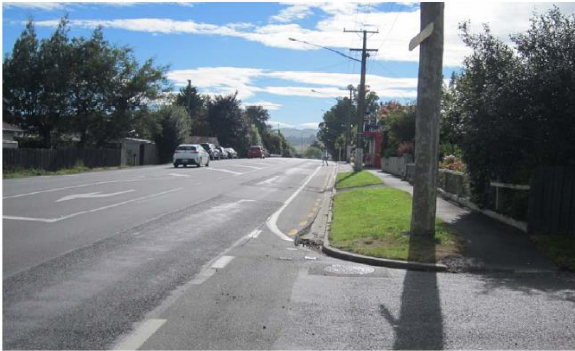
Figure 61. A view northeast along State Highway 1 at East Taieri township, showing the fan of Jaffray Stream. The road rises over the fan axis, and Jaffray Stream is conveyed in a culvert at the point where the road goes out of sight. If the culvert were to become blocked by debris during a major rainstorm, there is potential for flooding and sedimentation on the fan surface. Photo: D. Barrell, 17 February 2014, GNS Science.
