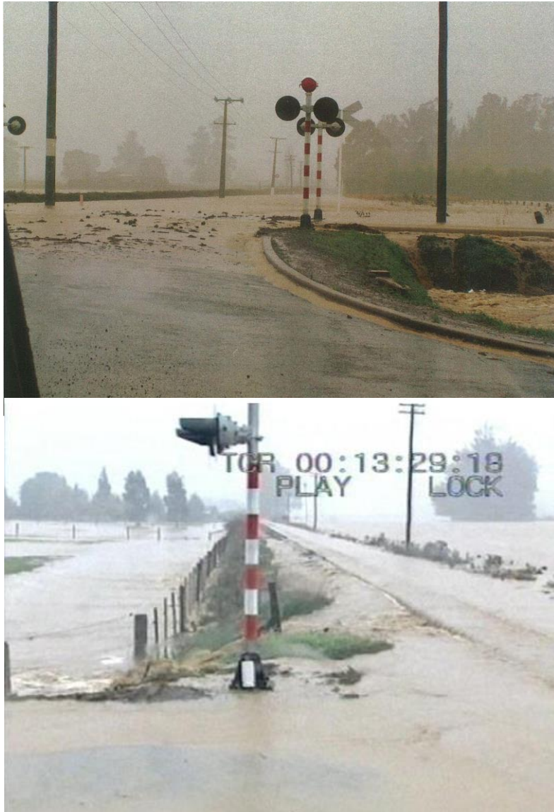
Figure 40. Water ponding behind the Taiari Gorge Railway, 26 April 2006
