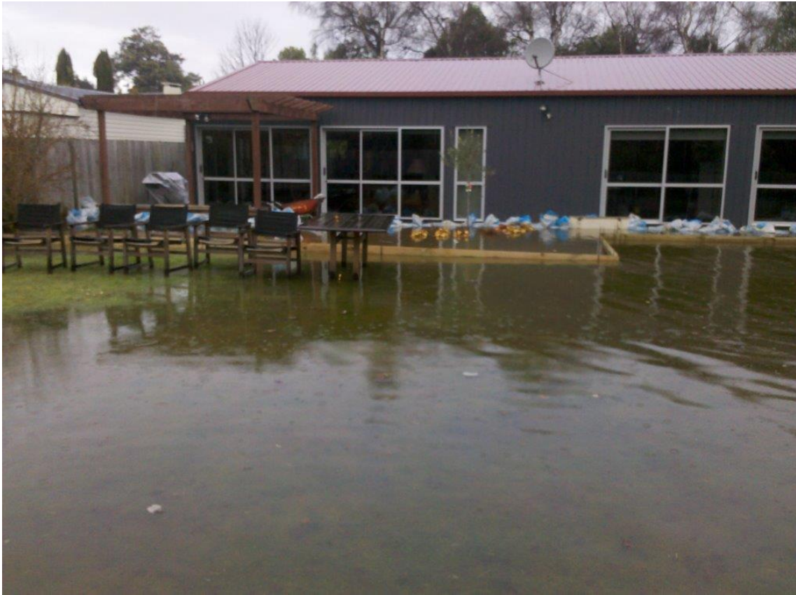
Figure 10. Water ponding around a residential property located within Area 1C, in July 2013
