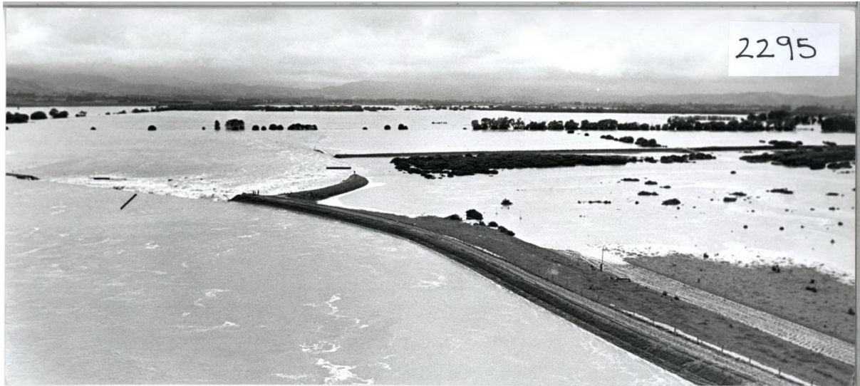
Figure 36. Breach of the northern section of the Area 13B ring bank during the December 1993 flood event. The location and direction of this photo is shown in Figure 33.
