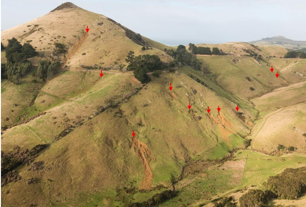
Figure 52. Aerial view of Harbour Cone, with landslide locations marked with red arrows, 16 June 2015
