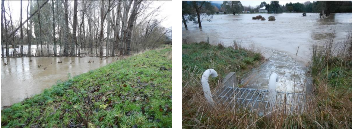
Figure 47. The floodbank (left) and pump station outlet (right) at Milton, downstream of SH1, 3 June 2015
