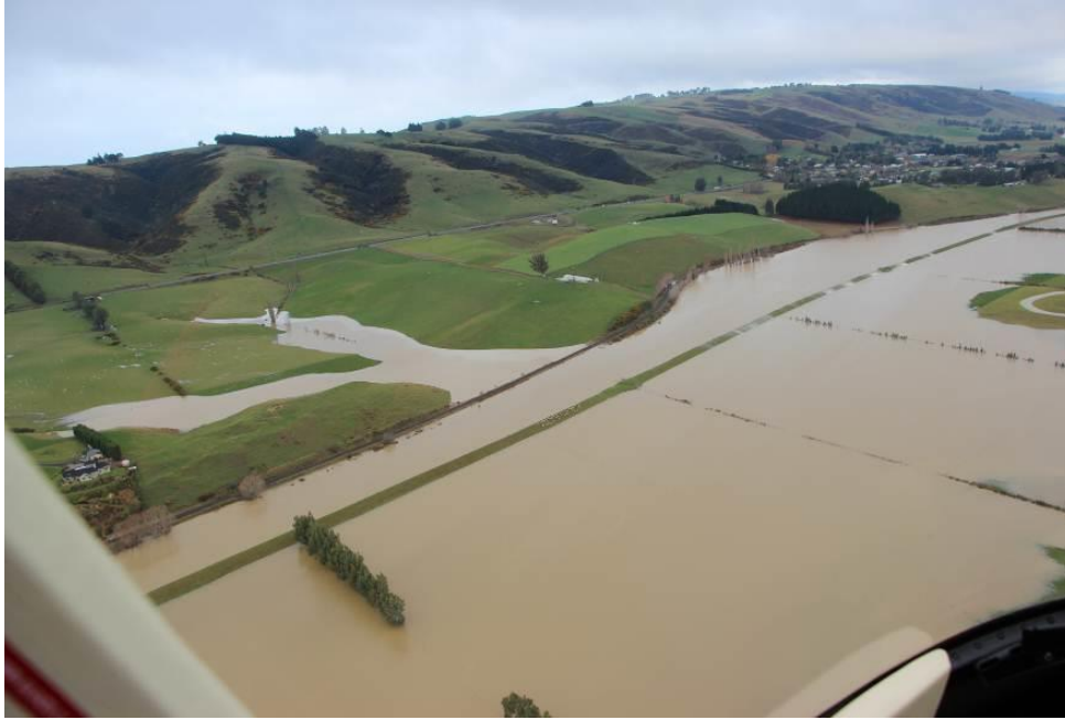
Figure 44. Ponding in the Lower Pond (note the overtopping of the Owhiro Stream true right bank) and at the flanks of the coastal hills – 4 June 2015
