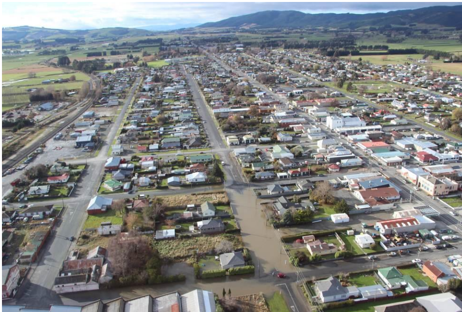
Figure 49. Aerial view of floodwater on Ajax Street (centre) Milton, with Union Street (SH1) to the right, 4 June 2015
