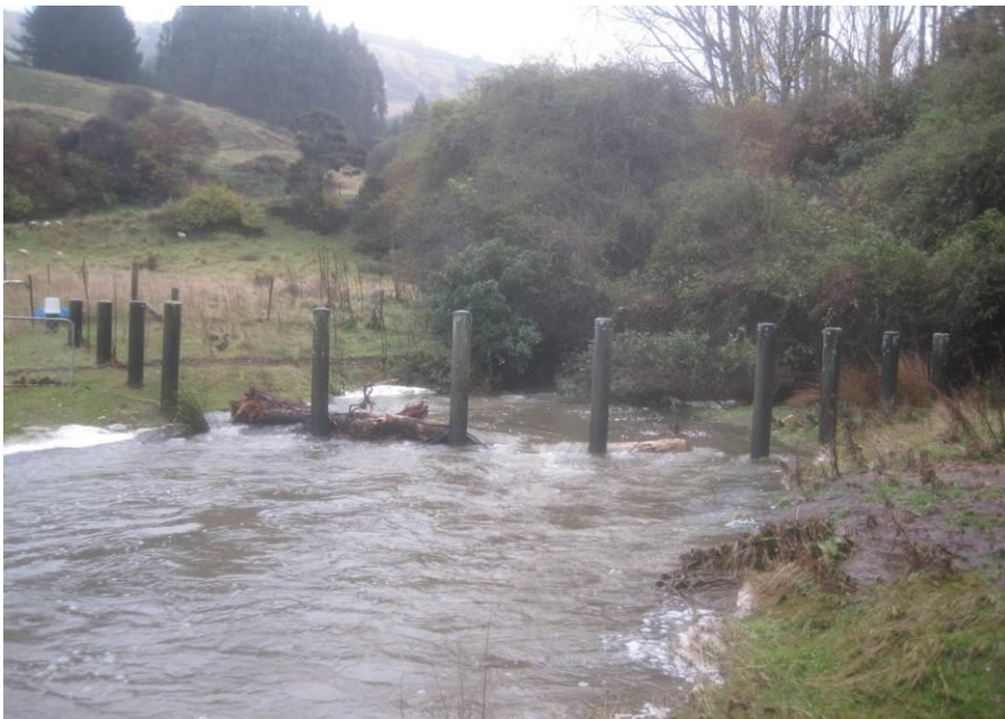
Figure 27. Lindsay Creek debris trap at Bethunes Gully during the event, 3 June 2015
