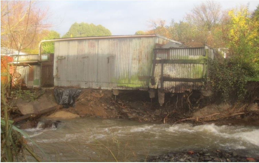
Figure 28. Bank erosion undermining a shed alongside Lindsay Creek at Kelvin Road, 4 June 2015
