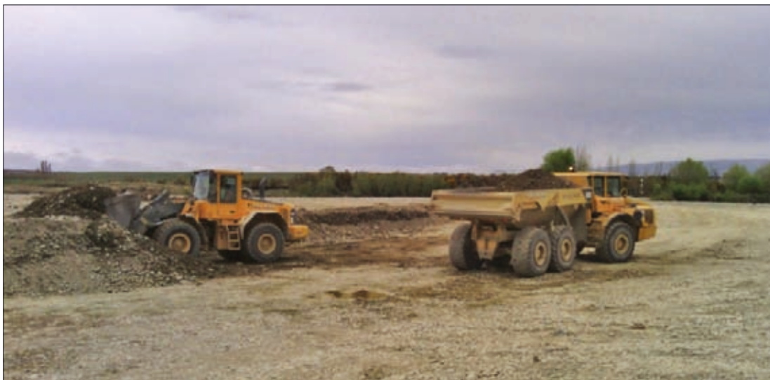
Figure 19. Gravel extraction in the Kauru River below the Kakanui Valley Road Bridge (November 2014)
