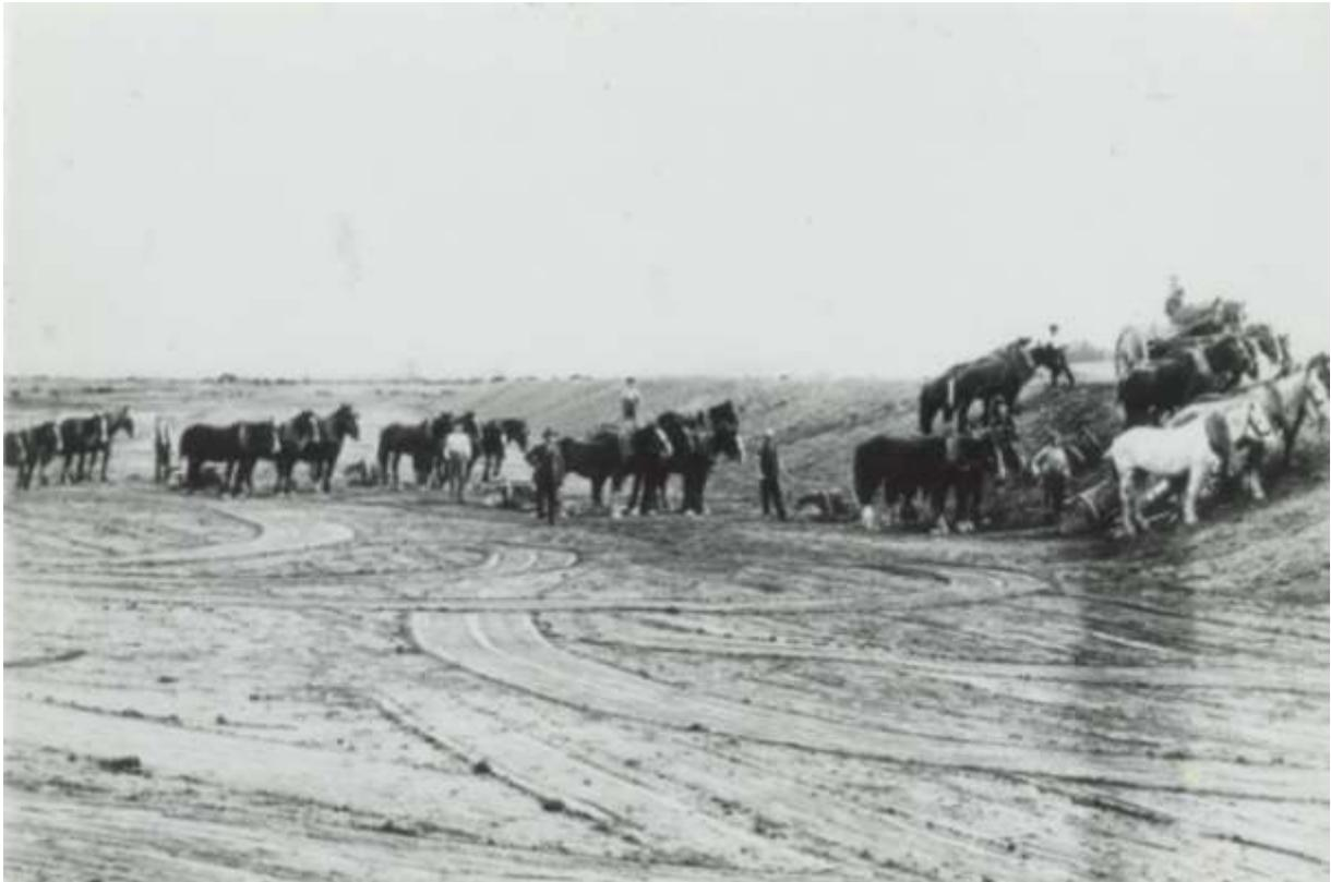
**Figure 2.4 Early construction of the Contour Channel on the West Taieri Plain (circa 1915).**
