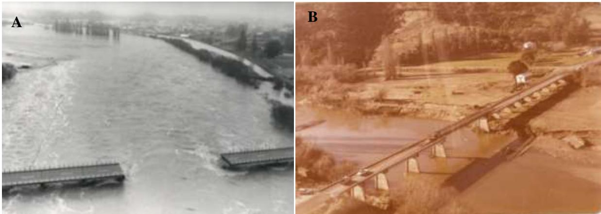
**Figure 2.9** A. Outram Bridge during the June 1980 flood (6 June at 3pm); B. Outram Bridge, with temporary Bailey bridge constructed post-event.
