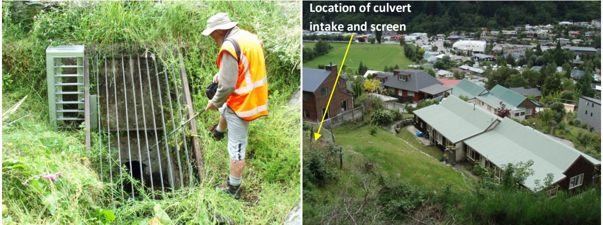
Figure 11.5 Reavers Lane alluvial-fan stormwater screen and culvert entrance (left). Residential properties at the head of the alluvial fan with respect to location of this structure (right)
