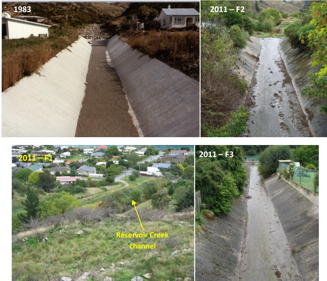
Figure 12.6 Reservoir Creek concrete-lined channel, upstream of SH 8 in March 1983 (top left), and in March 2011 (top right), looking upstream. Bottom left: Reservoir Creek channel upstream of concrete-lined channel. Bottom right: Reservoir Creek concrete-lined channel below SH 8
