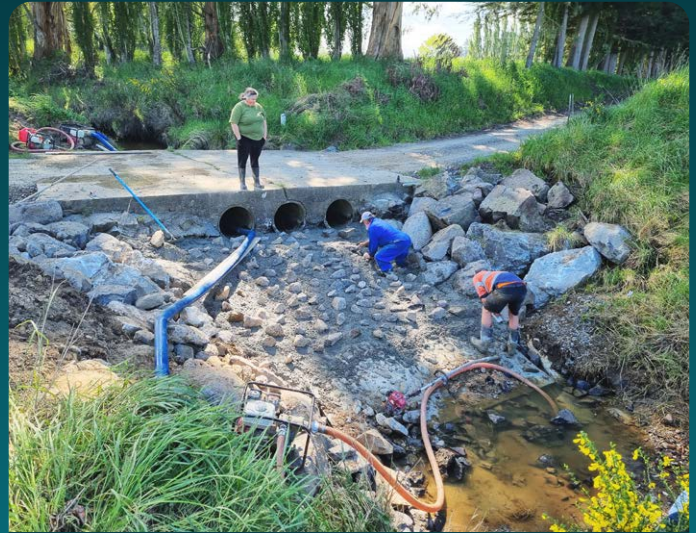
Figure 3. Construction of the rock ramp, showing the low-gradient ramp and rocks placed to reduce water velocity and provide resting areas for fish. © Matt Dale, Waterscape Connections
