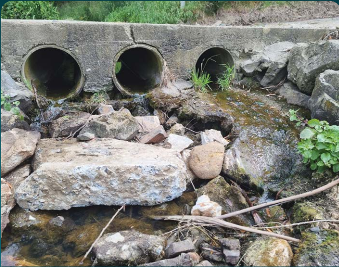
Figure 2. The downstream end of the Brooklands Road ford showing poor fish passage characteristics before construction of the rock ramp. © Matt Dale, Waterscape Connections
