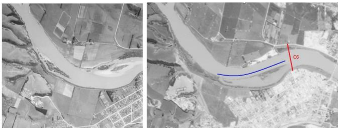
Figure 6-1: Aerial photographs from 1946 (left) and in 1995 (right). Blue line indicates the mid-channel river training works upstream of cross-section C6.
