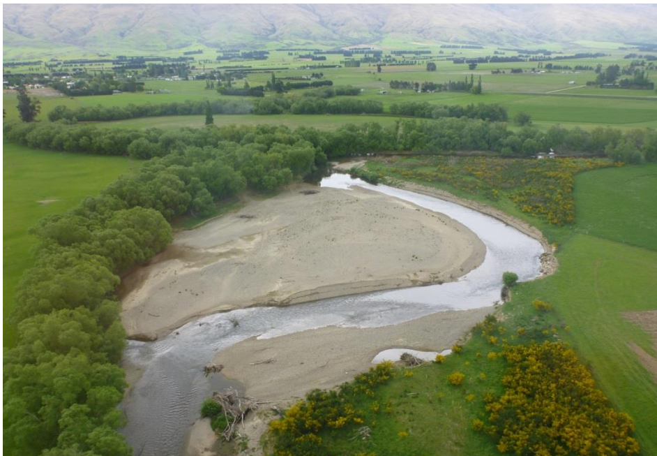
Bank erosion, in the Taieri River (November 2015)
