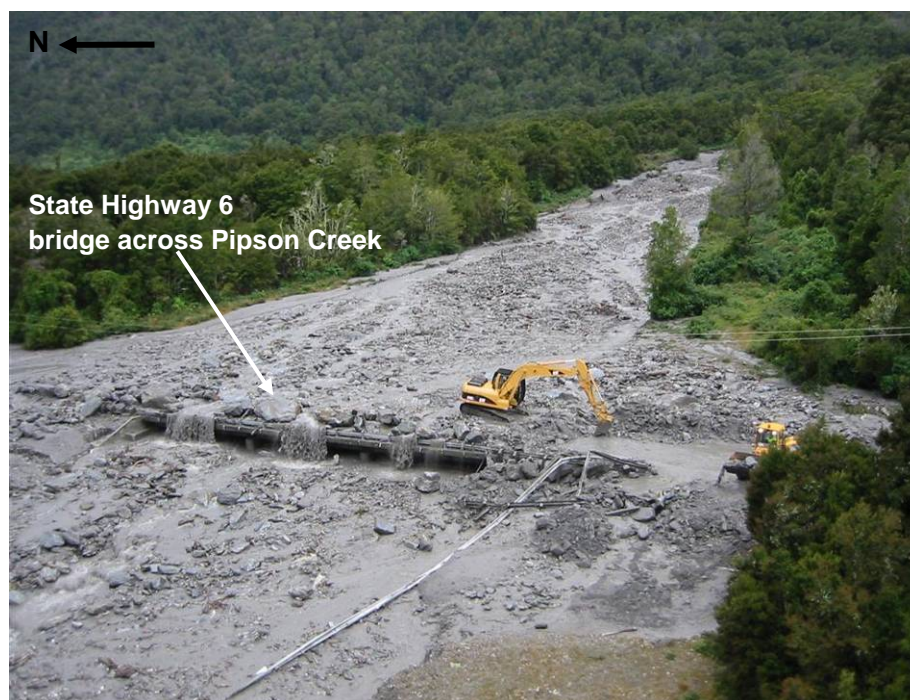
Figure 4: Photograph showing debris flow clean up work on SH6 at Pipson Creek. Photograph taken 10 th March 2004.
