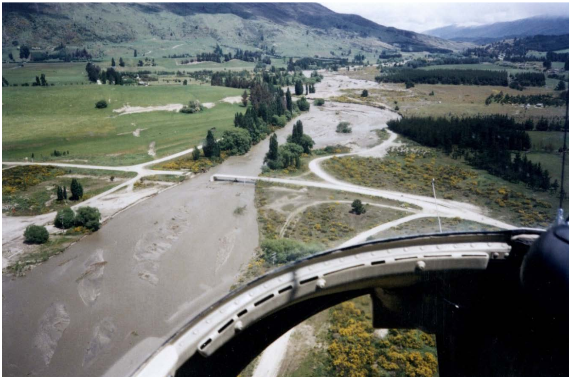
Figure 12. Ballantyne Road bridge (Cardrona River), looking upstream (photography taken after the peak of the flood, November 1999)
