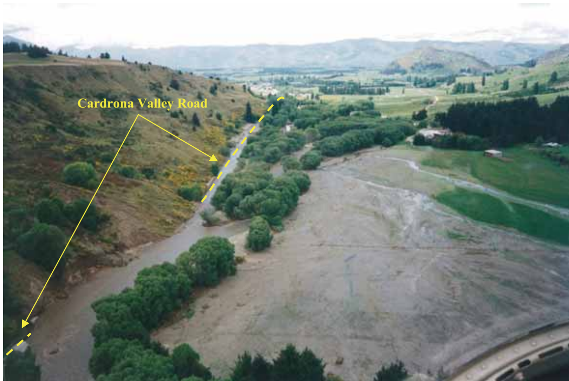
Figure 4.2 True left bank erosion of the Cardrona Valley Road near The Larches, November 1999
