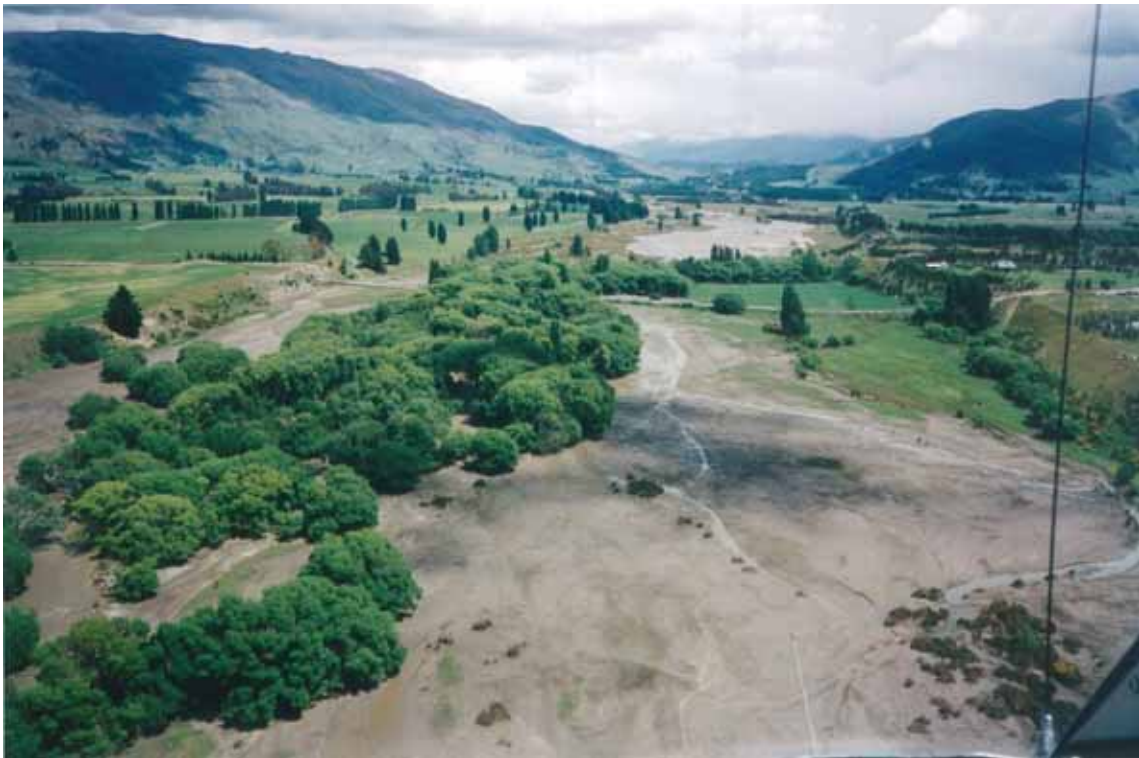
Figure B.15 Flood sedimentation below the State Highway 6 Bridge looking upstream, November 1999
