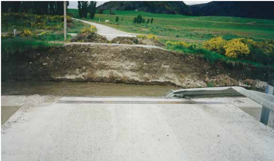
Figure 4.5 True right bank approach of the Ballantyne Road bridge following November 1999 flooding
