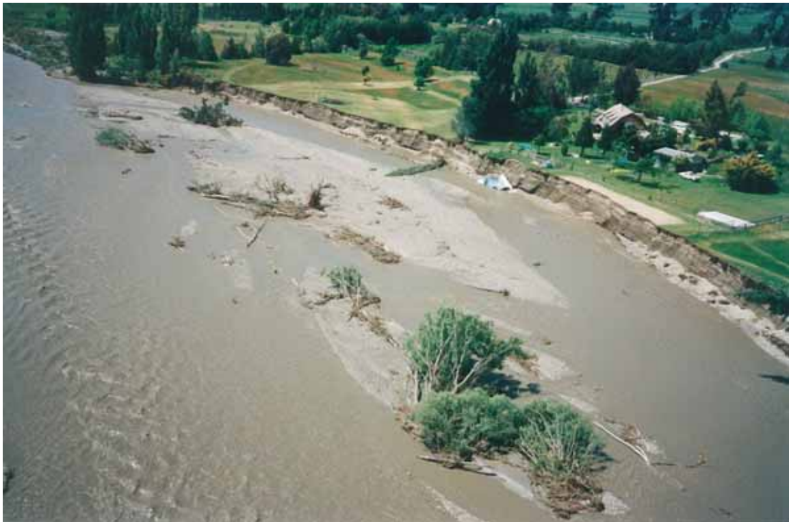
Figure B.11 True right bank erosion downstream of The Larches and upstream of the Ballantyne Bridge looking downstream, November 1999
