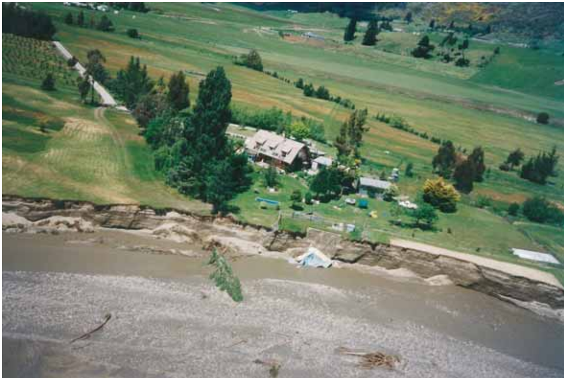
Figure 4.4 True right bank erosion downstream of The Larches, November 1999
