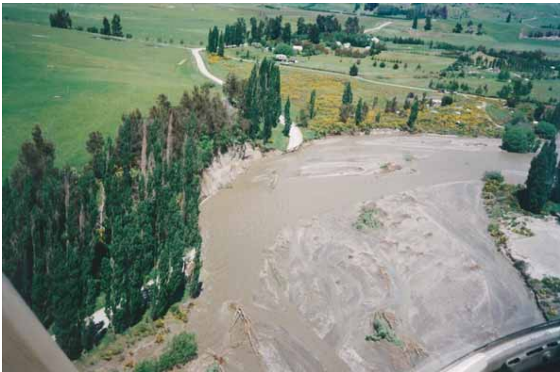
Figure B.12 True right bank erosion downstream of The Larches and upstream of the Ballantyne Bridge looking upstream, November 1999
