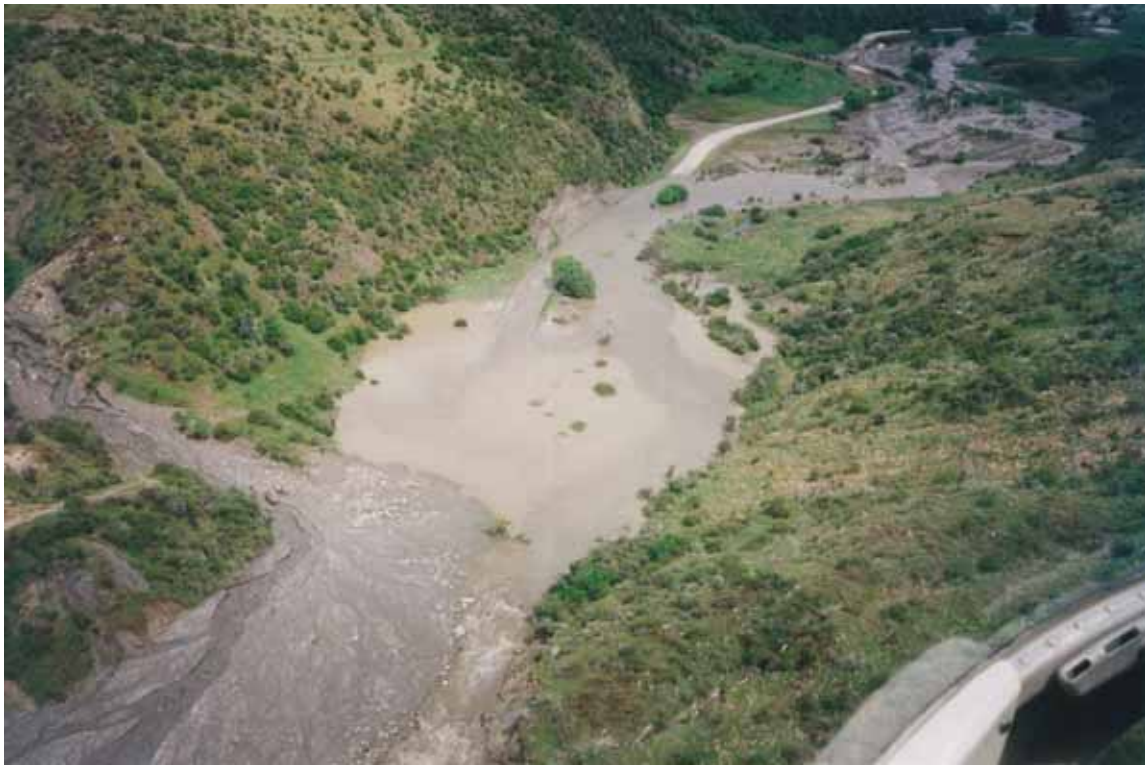
Figure B.3 Debris dam formed over the Cardrona Valley Road in the upper valley reaches looking upstream, November 1999
