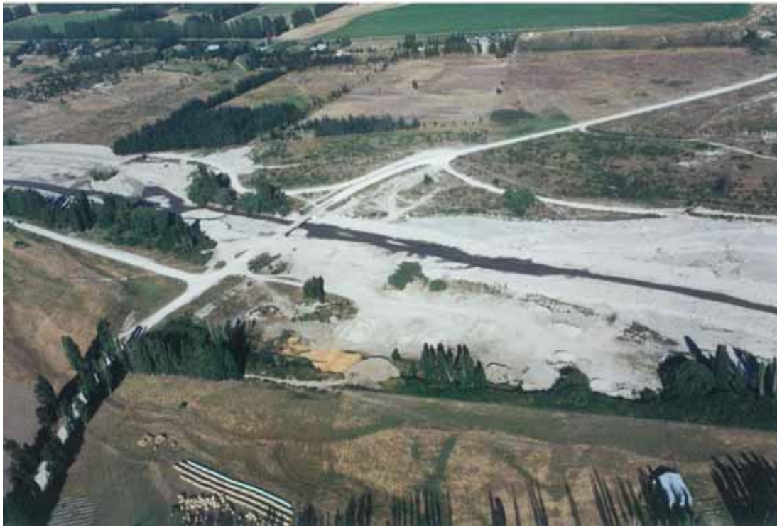
Figure 5.2 Ballantyne Road Bridge on 14 January 2000. Artificial embankments are evident along each side of the Cardrona River; part of the post-November 1999 remedial works
