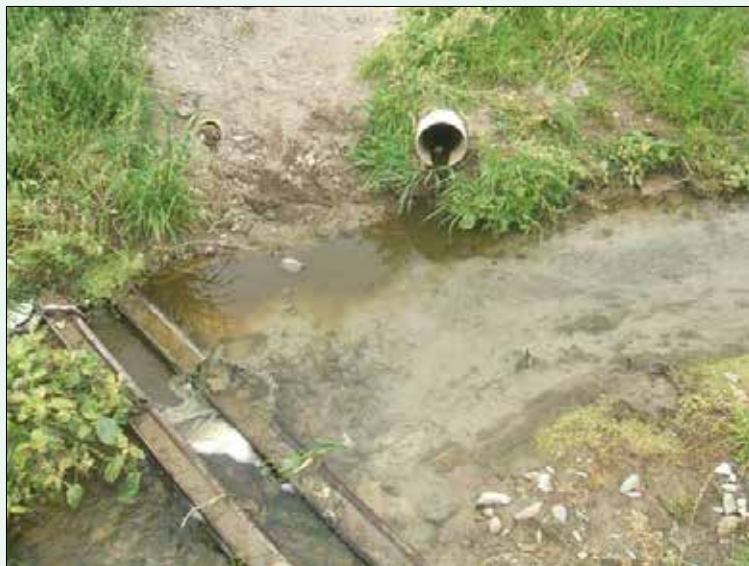
Tiles running green like this are a sure sign that effluent is being applied poorly. Where there are tile drains, make sure that the timing and application rate of effluent is carefully managed.
