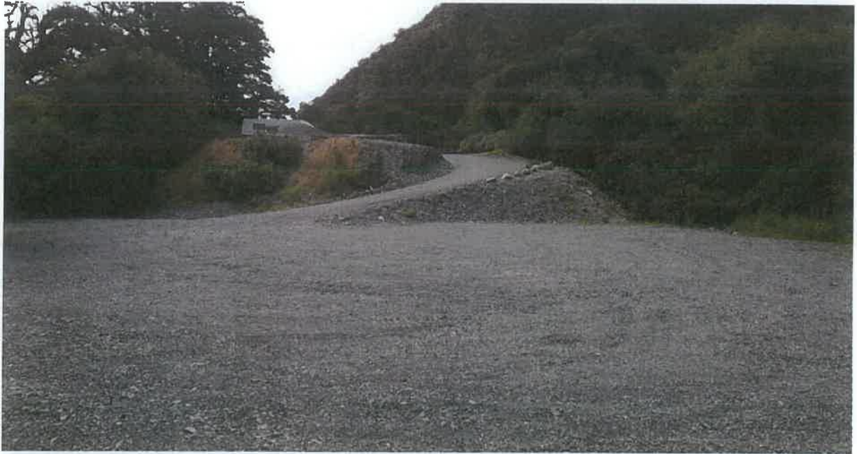
Figures 3 and 4 - extensions to the extensions to the original car park
