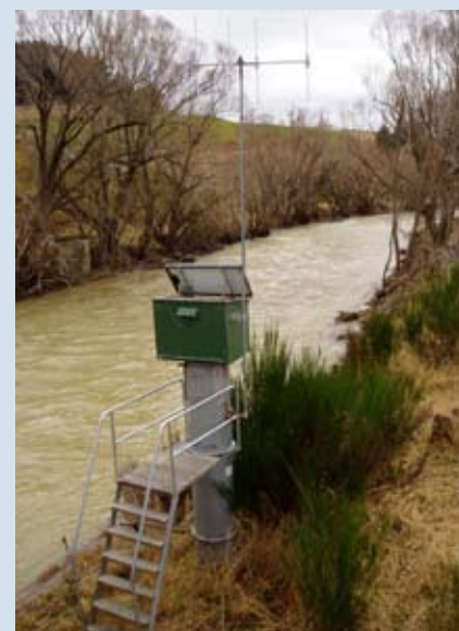
Flow monitoring station at Tiroiti
