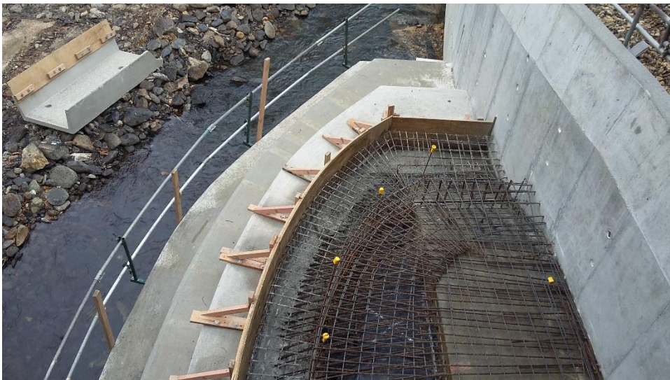
Figure 5: Construction of walls and terraces upstream of and beneath the Information Technology Services (ITS) building (north side of channel).
