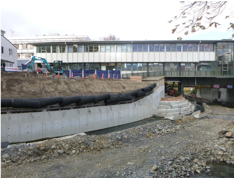
Figure 4: Construction of walls and terraces upstream of and beneath the Information Technology Services (ITS) building (north side of channel).
