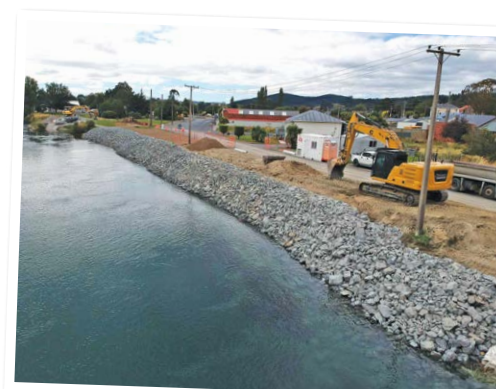
Floodbank repair in Kaitangata
