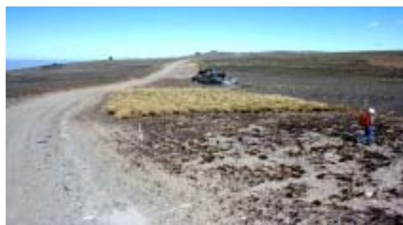
Figure 25: View south along the crest of the Old Man Range at 1600m, showing an area (20m x 40m) with 800 narrow-leaved snow tussocks (sourced at 1220m), planted early in 1975, following the 'blading' of a 20m-wide strip alongside the road constructed to Obelisk in late 1974 for a TV translator. Feb., 1982.
