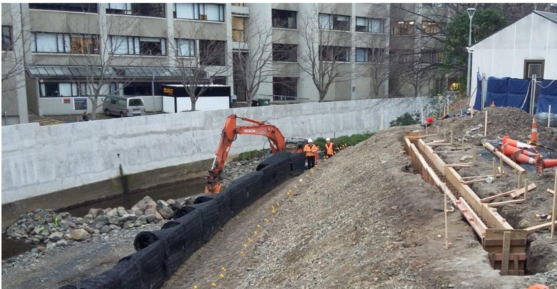
Figure 2: Construction of ground beam to support cellular confinement to enable landscape planting and balustrade on left bank upstream of the Information Technology Services (ITS) building.
