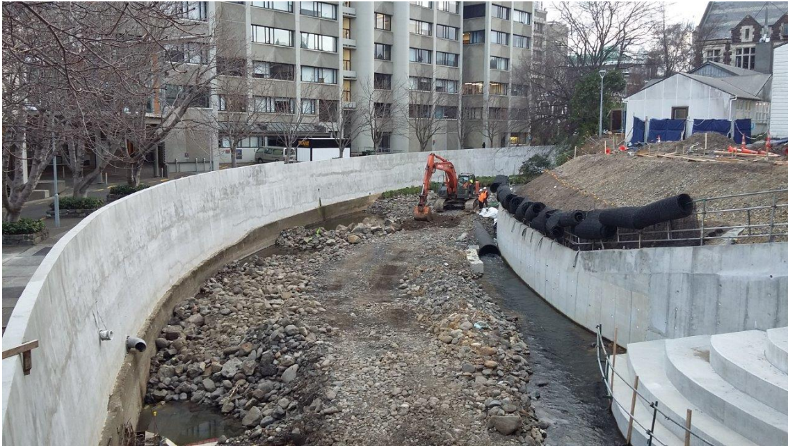
Figure 1: Construction of walls and terraces upstream of the Information Technology Services (ITS) building.
