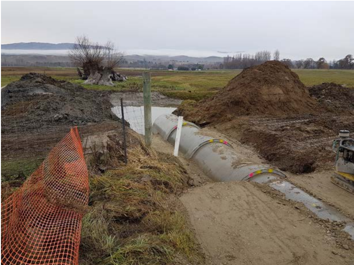
Figure 6: Culvert pipes installed on Stock Truck Effluent Disposal Site access road along SH85.
