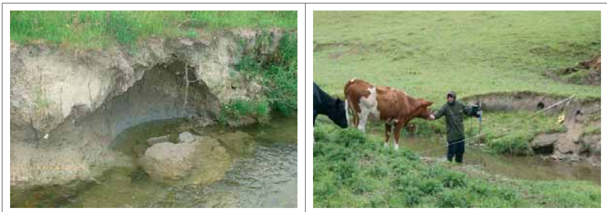
Figure E-1: Stock access and bank slumping/collapse.
