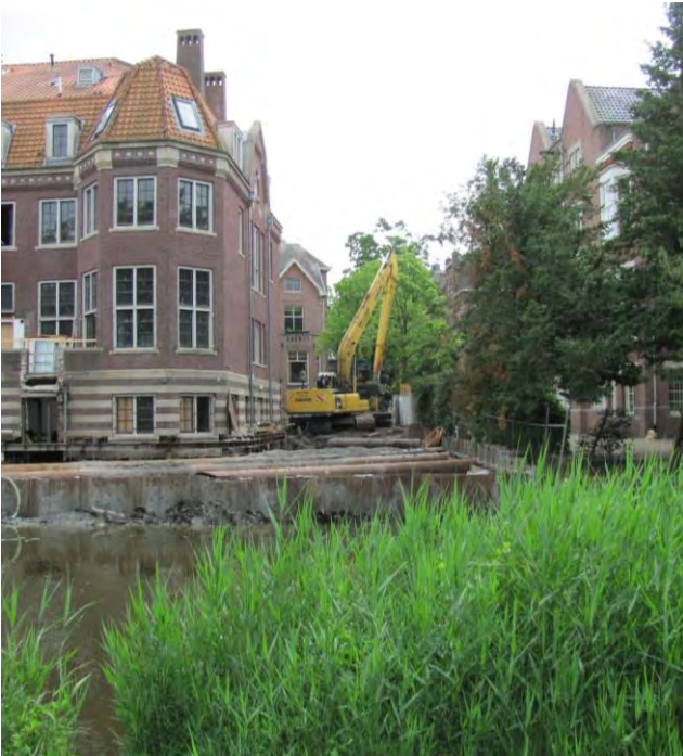
Figure 20: Canals and restoration construction being undertaken, Vondel Park (Amsterdam).
