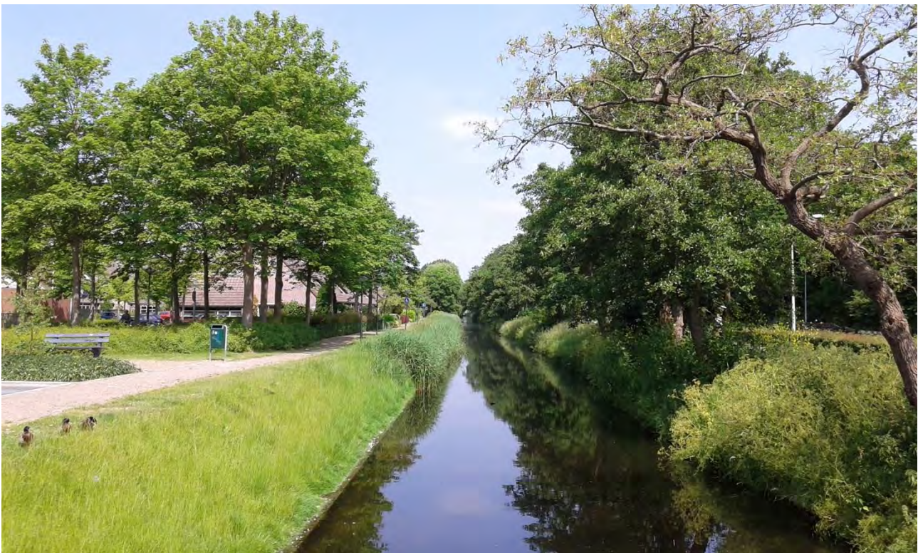
Figure 30: Pumped open canal in Hoorn, The Netherlands.
