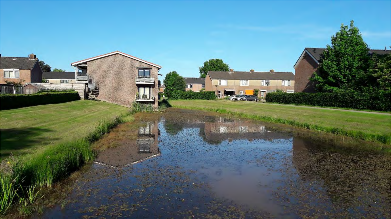
Figure 25: New open canal dug during the district renovation of Oosterwolde-Zuid: water storage, drainage, improved water quality and overall quality of the public space.
