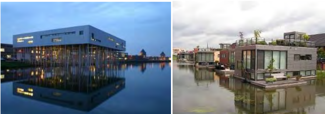
Figure 7: Examples of waterproof buildings (left: pile house; right: floating house).
