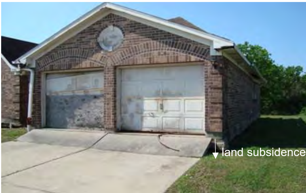
Figure 22: Land subsidence in New Orleans - land has subsided but not the floor level.
