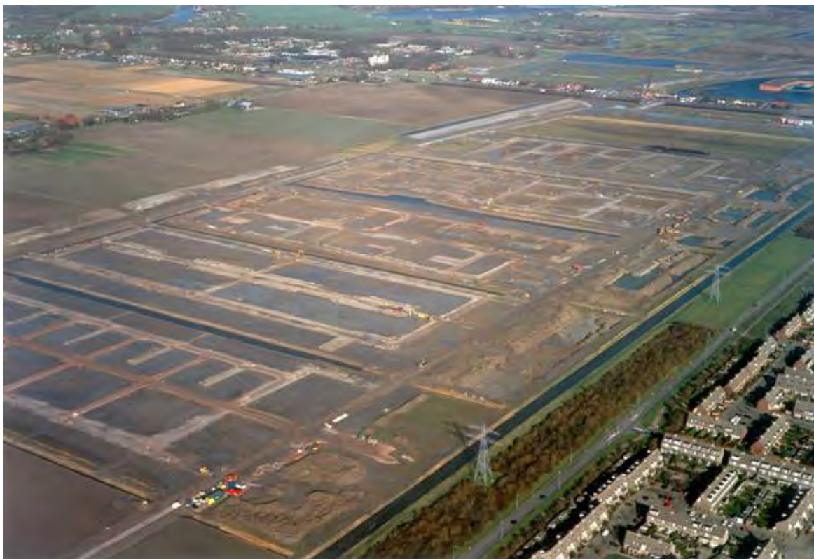
Figure 5: Excavation filling in progress for a new urban development The Netherlands, photograph supplied by Deltares.
