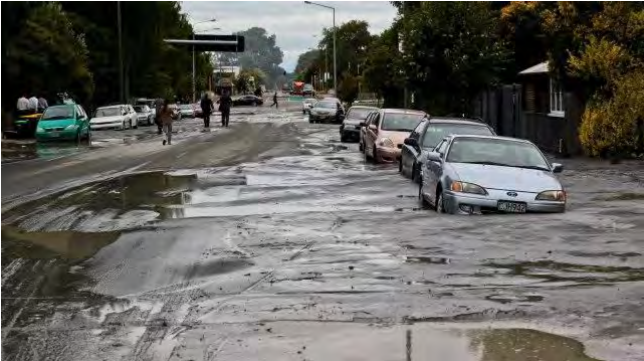
Figure 29: Effects of liquefaction on Killmore St (Asher Trafford), Christchurch, following the Canterbury earthquakes (source: https://keithwoodford.wordpress.com/2011/02/27/understanding-the-christchurch-earthquake-building-damage/ ).
