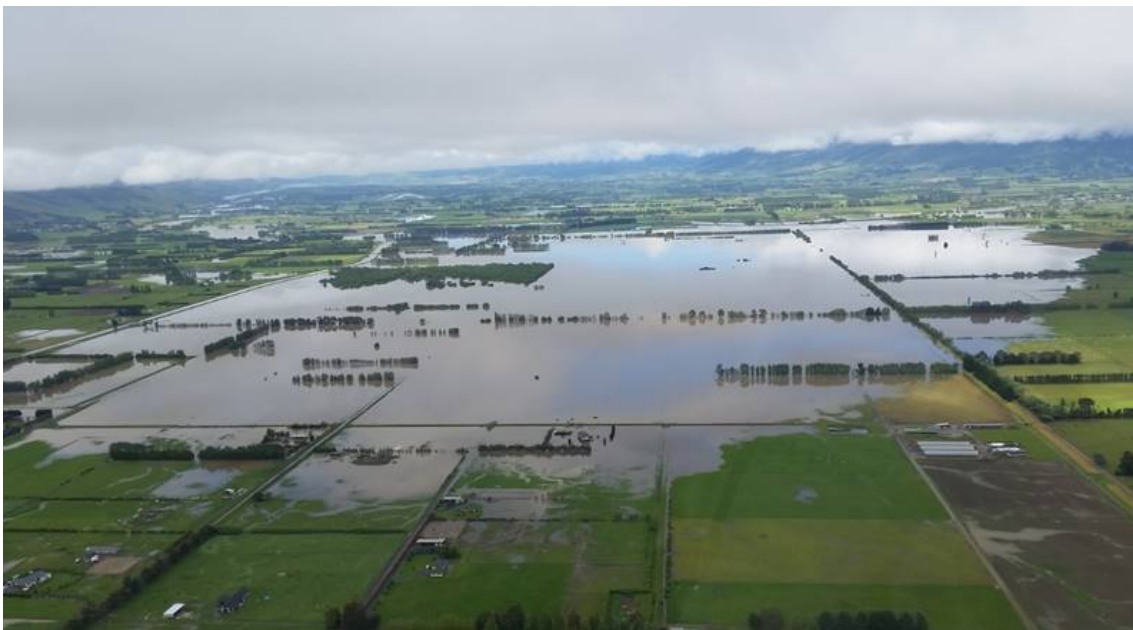
Figure 4. Looking south to the East Taieri Upper Pond (Lower Taieri Flood Protection Scheme) at 0945hrs on 22 November 2018. The pond had just reached its maximum height and volume for this event, to date (approximately 29 million cubic metres of water). The Taieri River and Riverside Spillway (Figure 3) are at the far end of the pond.
