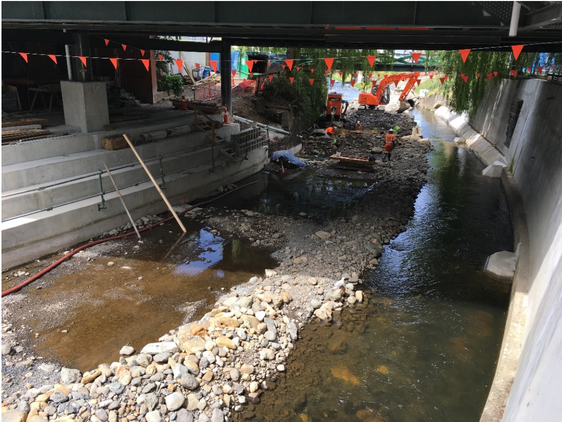
Figure 9. Looking downstream along the bed of the Water of Leith under the Information Technology Services (ITS) Building (14 November 2018). Work is taking place on the last of the instream weirs.
