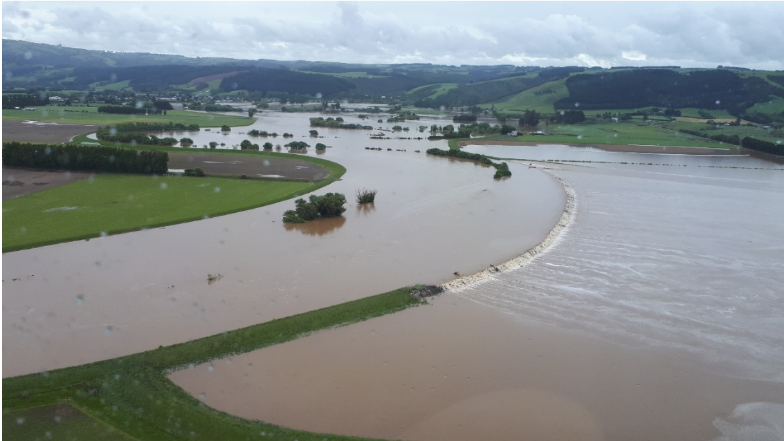
Figure 3. Riverside Spillway (Lower Taieri Flood Protection Scheme) at 1052hrs on 21 November 2018. Water is flowing into the East Taieri Upper Pond at right. The Taieri River (at left) was flowing at approximately 900m 3 /s, after peaking at 1,400m 3 /s approximately 11 hours earlier.
