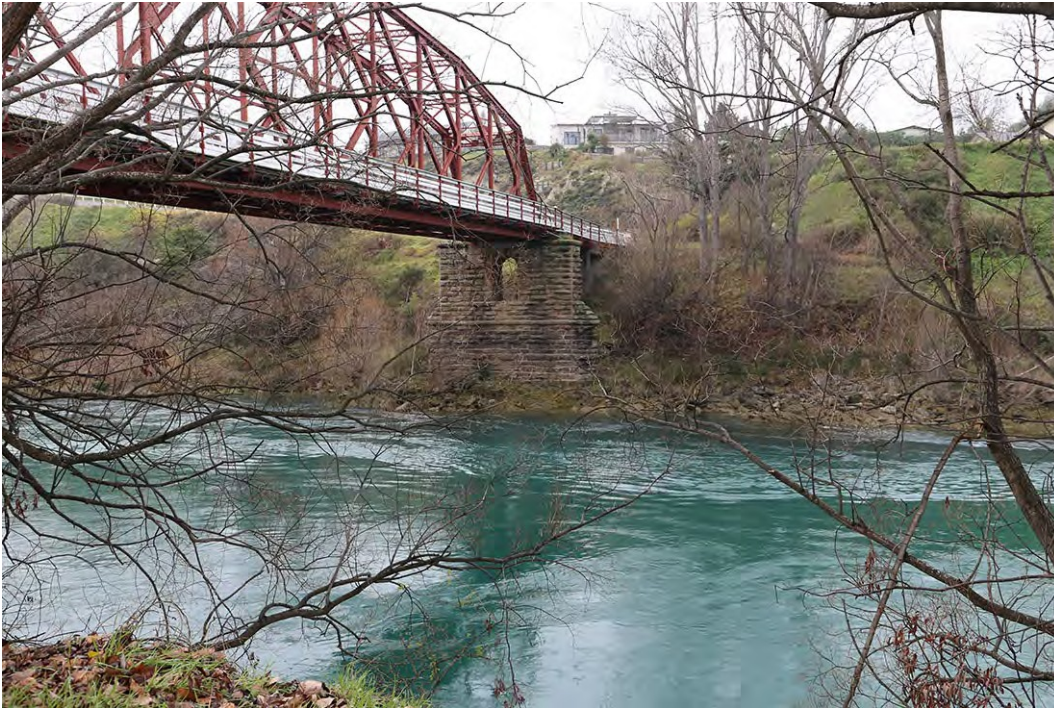
Flowing under the historic bridge at Clyde - river flows in this reach are regulated by the Clyde Dam upstream.
