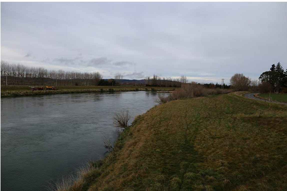
Matau Branch of the river at Stirling bridge - the lower reaches of the river flow across flat land and old floodplains, largely contained by stopbanks and lined with willow.
