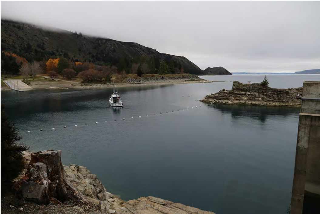
Lake Hāwea control gate - Lake Hāwea levels can fluctuate by up to 8.0 m resulting in changing exposure of the shoreline
