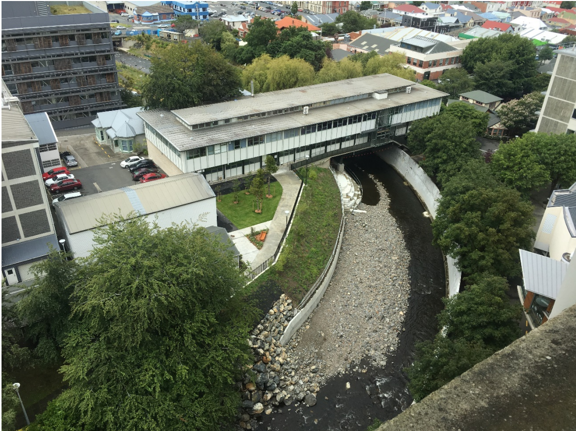
Figure 6. Water of Leith looking downstream towards the University of Otago Information Technology Services (ITS) Building (20 December 2018).
