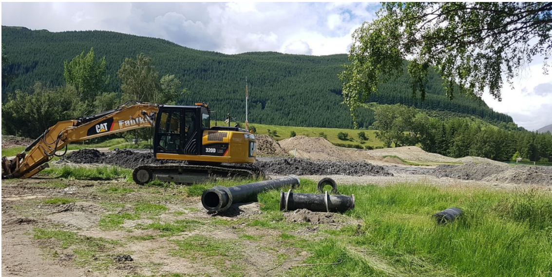
Figure 1. Contractors preparing to install the outfall structure that could discharge Arrow Irrigation Scheme water into Hayes Creek, Arrowtown (14 December 2018).
