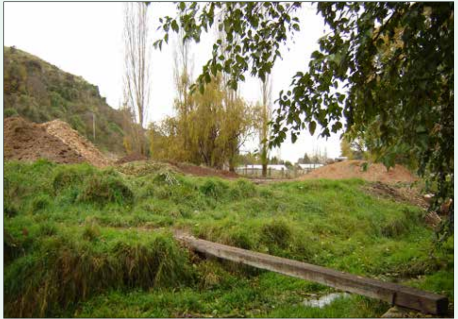
Compost heap leaching to a waterway. This is prohibited.
