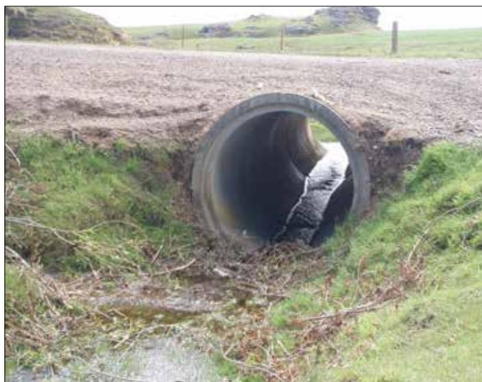
This culvert provides fish passage but has no measure to stop animal waste runoff to the stream.
