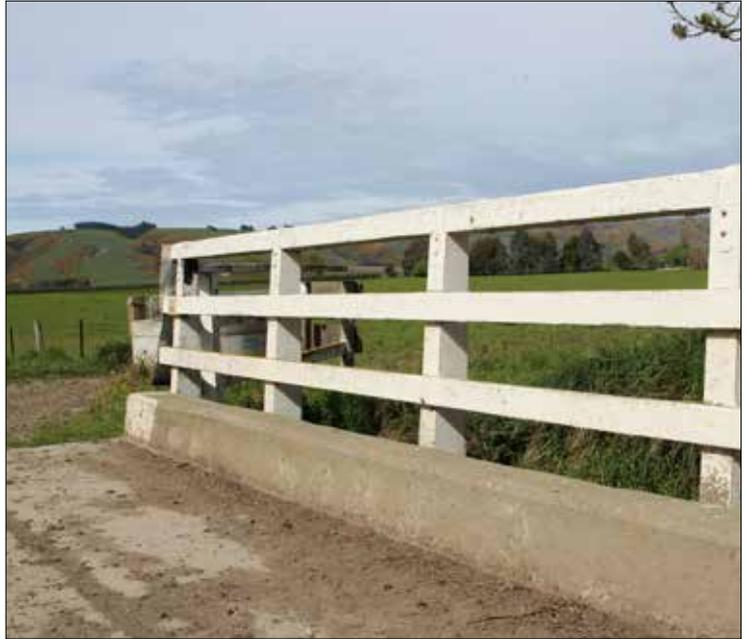
The raised edges on this bridge prevent effluent washing into the stream. It is a good idea to extend the kerbs beyond the length of the bridge to channel runoff towards the paddock and not into the waterway.
