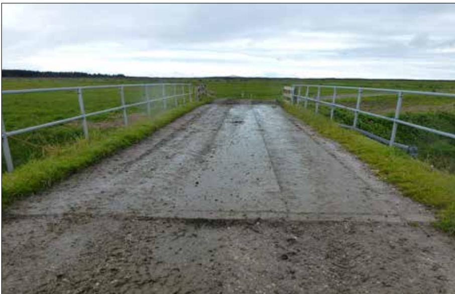
This is a good example of a well-designed bridge with a raised lip on the side and slightly raised approaches to direct runoff away from the waterway.
