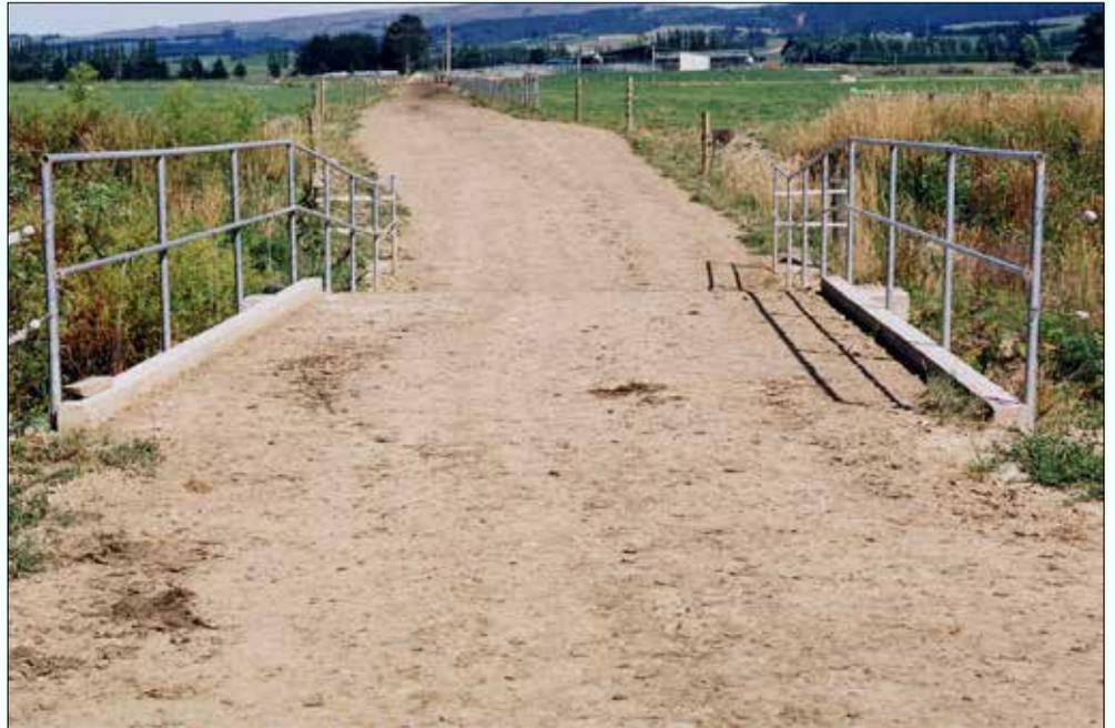
This bridge is designed to stop runoff from entering the waterway by installing a kerb on the side and maintaining a large a vegetation buffer. Contour the deck to direct runoff away from waterways.
