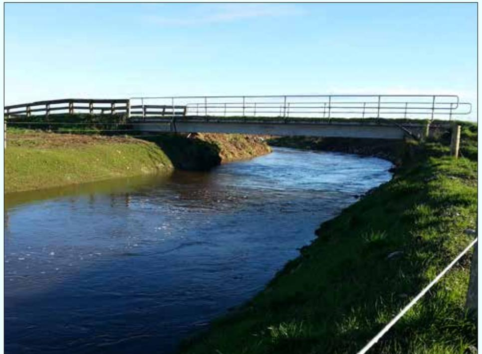
A stock crossing designed to prevent mud and animal waste getting into the water. Drainage flows need to be dispersed and filtered over vegetation before reaching the waterway.
