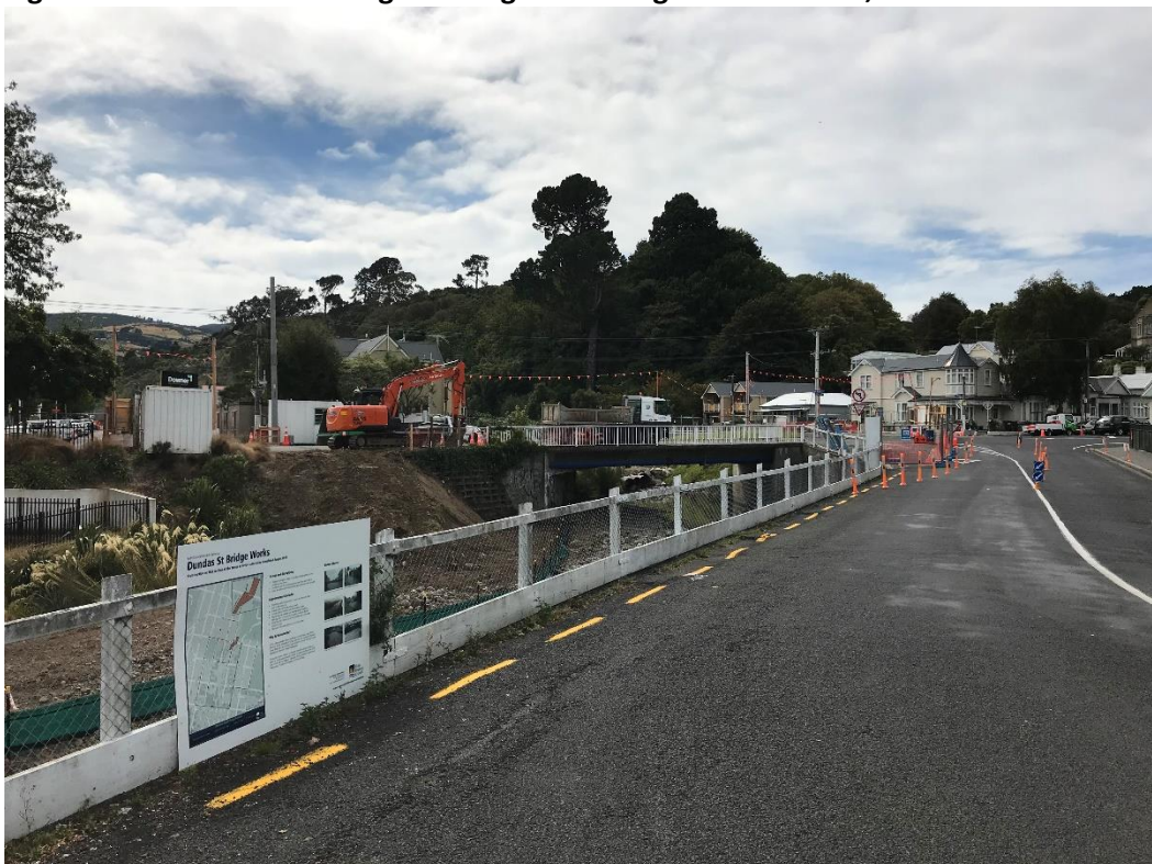
Figure 5: Water of Leith looking upstream to Dundas Street bridge, 7 March 2019
