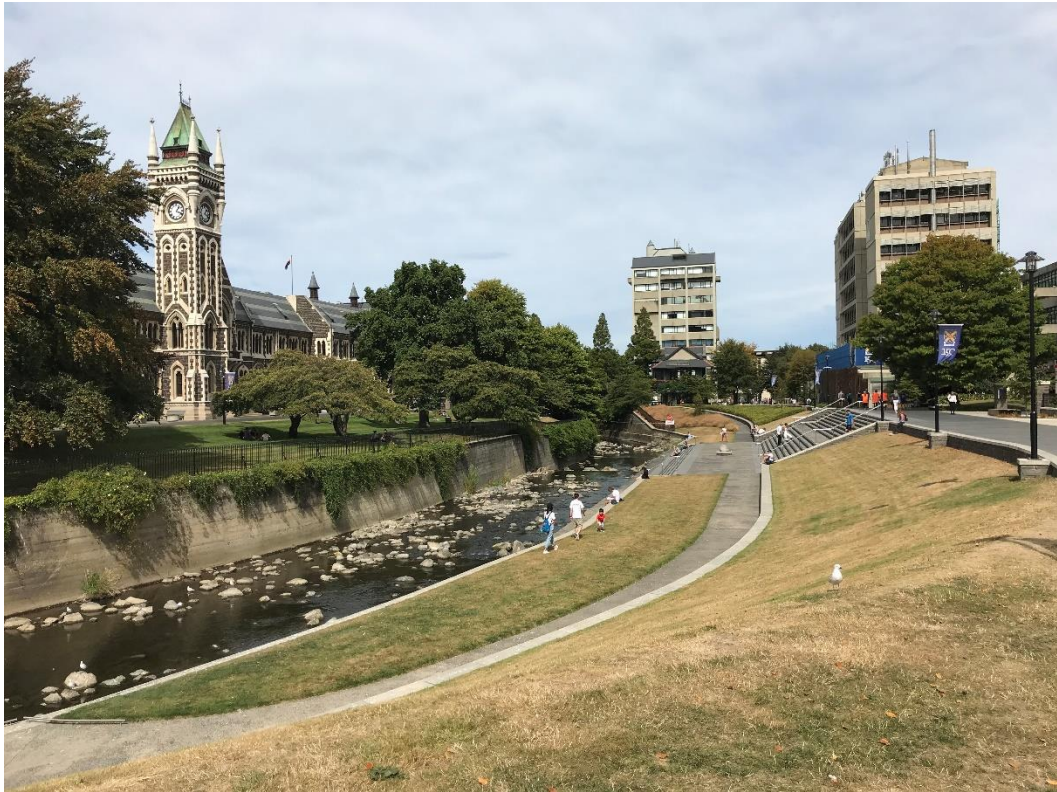
Figure 6: Leith Flood Protection Scheme outside University of Otago Registry Building 7 th March 2019
