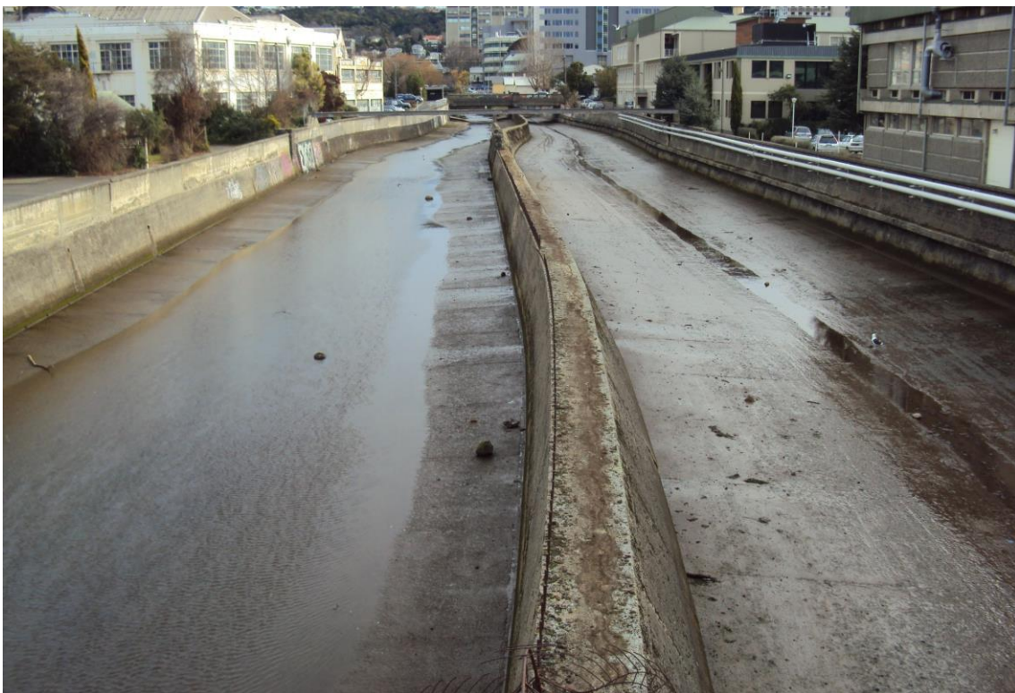
Figure 5: Anzac Avenue Bridge looking upstream towards Forth Street November 2017.
