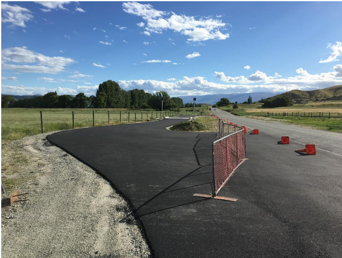
Figure 1: SH85 near Brassknocker Road
