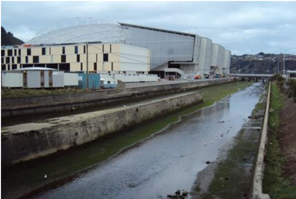
Figure 2: Anzac Avenue Bridge to State Highway 88 before installation of weirs in July 2011
