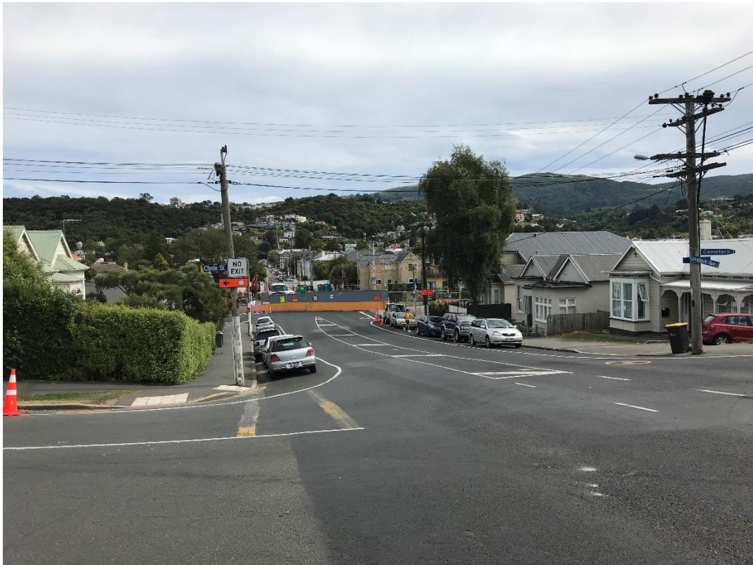
Figure 4: Dundas Street bridge looking west along Dundas Street, 7 March 2019
