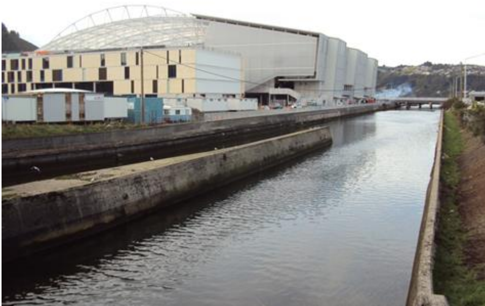
Figure 3: Anzac Avenue Bridge to State Highway 88 with weirs in place in October 2011.
