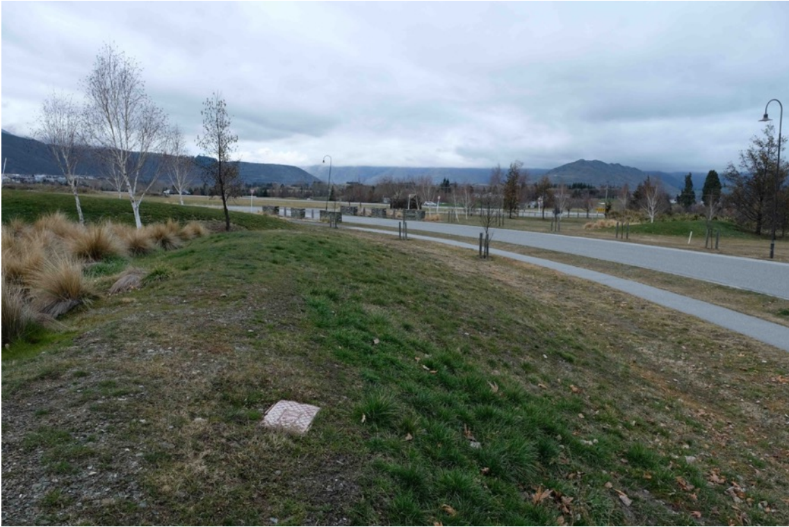
Figure 43 Pump station 20 beside Essex Avenue, Arrow Town.
