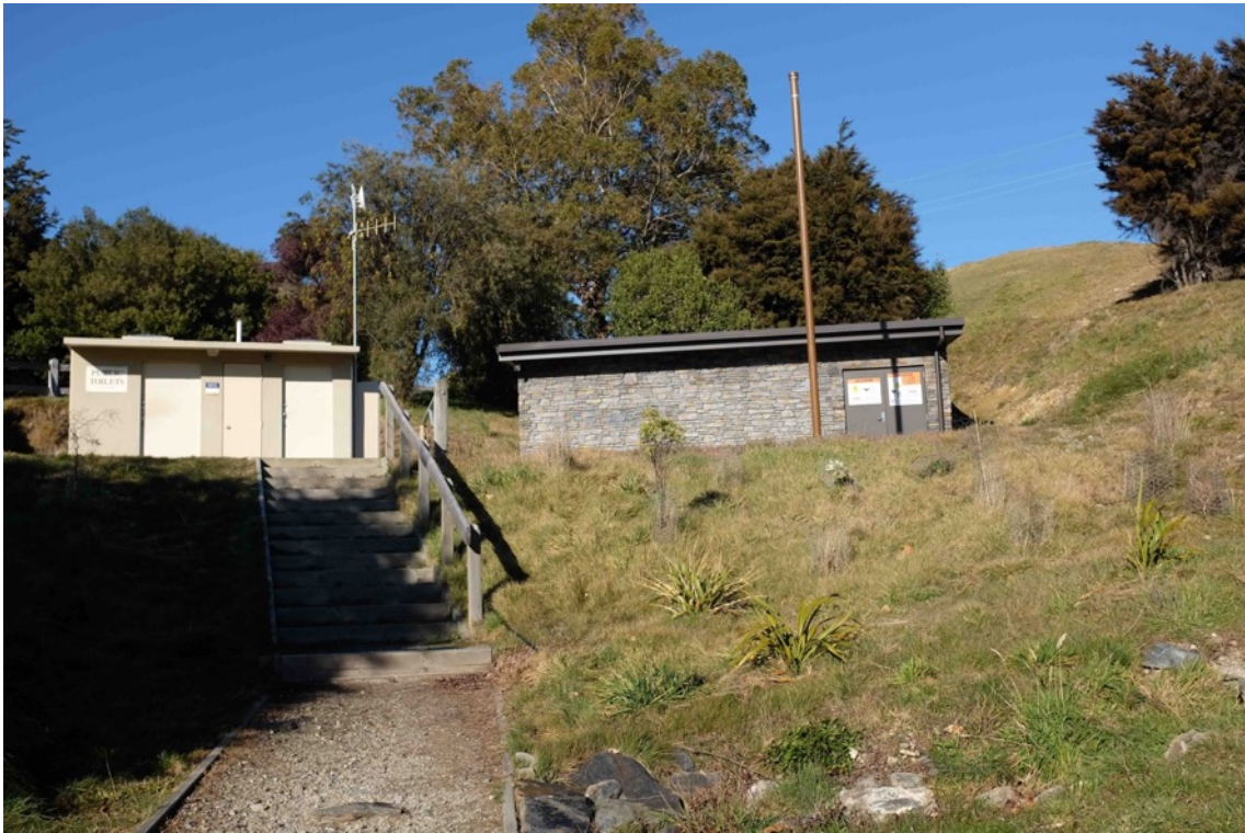
Figure 62 Pump Station 33 on Scotts Beach Road on the shore of Lake Hāwea.
