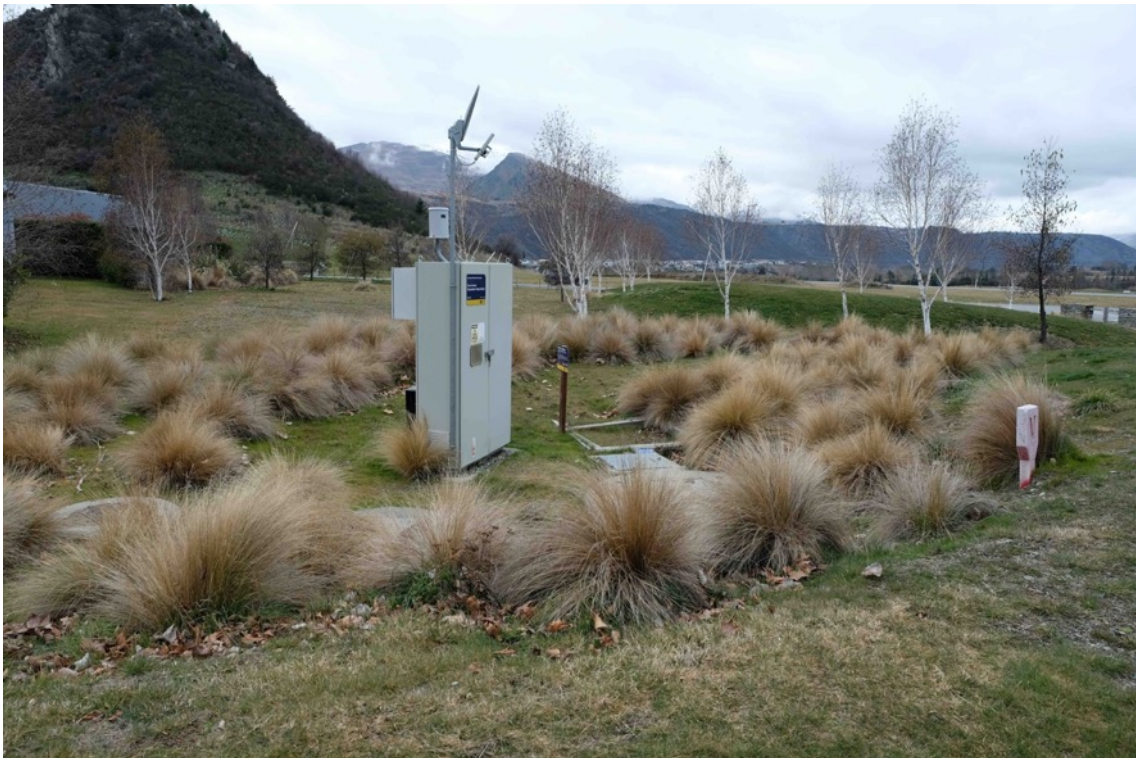
Figure 42 Pump station 20 beside Essex Avenue, Arrow Town.
