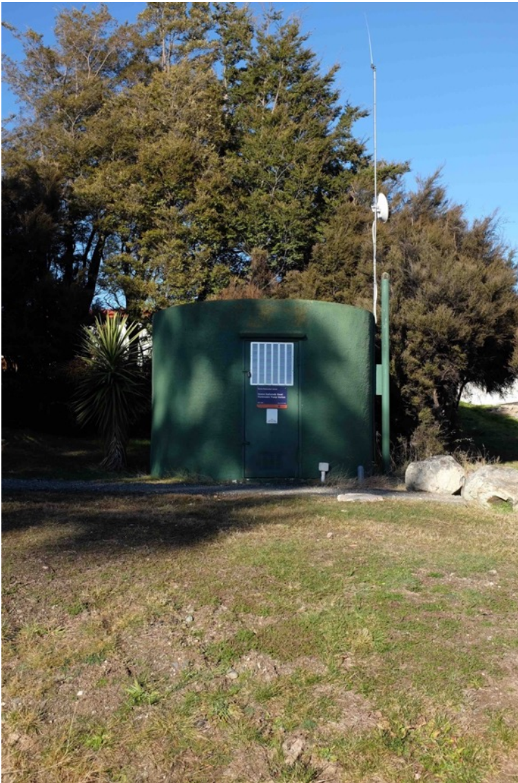
Figure 60 Pump Station 32 on Hāwea esplanade track on the shore of Lake Hāwea.
