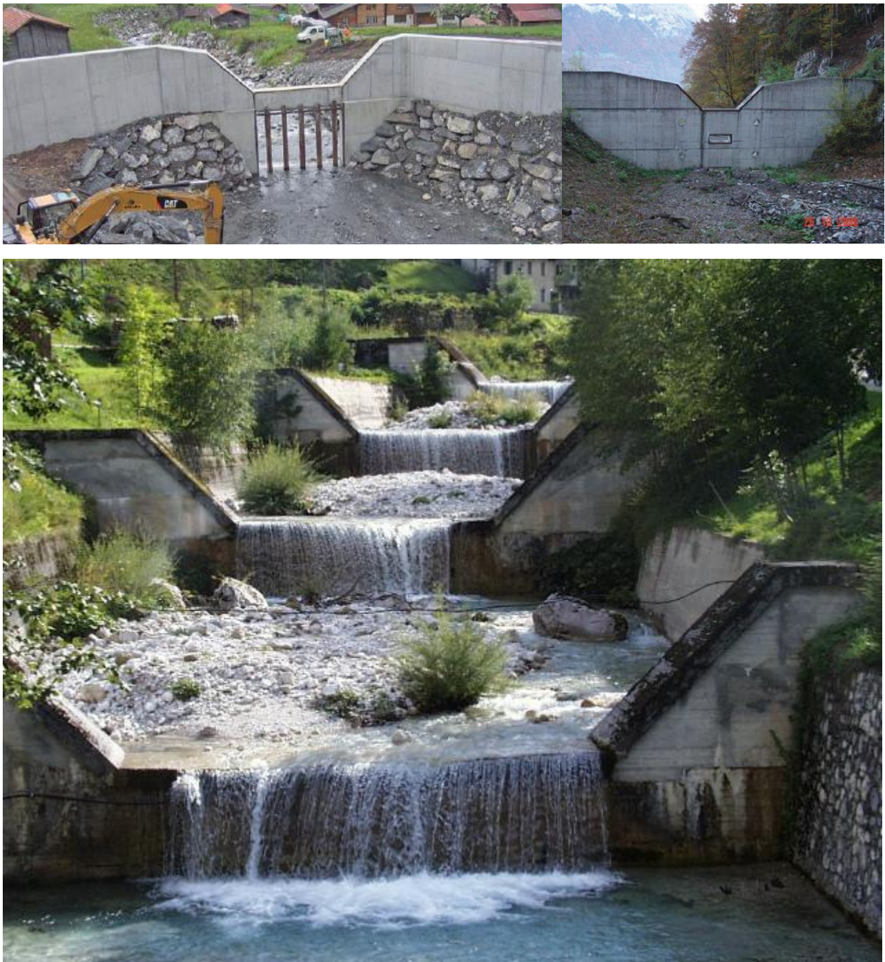
Figure 1: top left: concrete retention structure with central steel rake to separate debris material from water (source: Herzog Ingenieure, Davos, Switzerland); top right: concrete sediment retention structure in Switzerland (source: (Wendeler, 2016)); bottom: series of check dams in European Alps (Comiti, Lenzi, & Mao, 2013).
