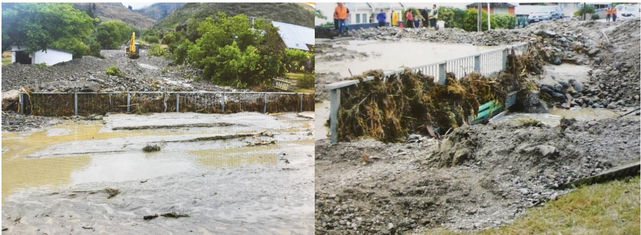
Figure 16: Aggradation of debris above SH8 crossing and avulsion of water and fine debris on 26 November 2017 (source: Withington, Teviot Valley Tempest, 2018).
