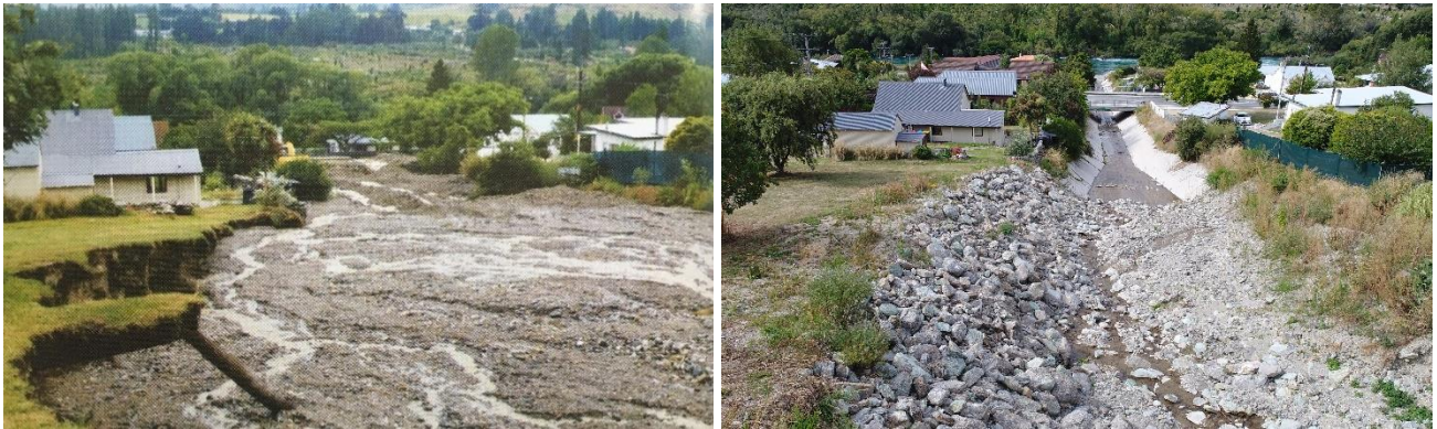
Figure 15: left: Aggradation of debris at entrance to concrete channel after 26 November 2017 event (source: Withington, Teviot Valley Tempest, 2018); right: Channel status 26 February 2019.
