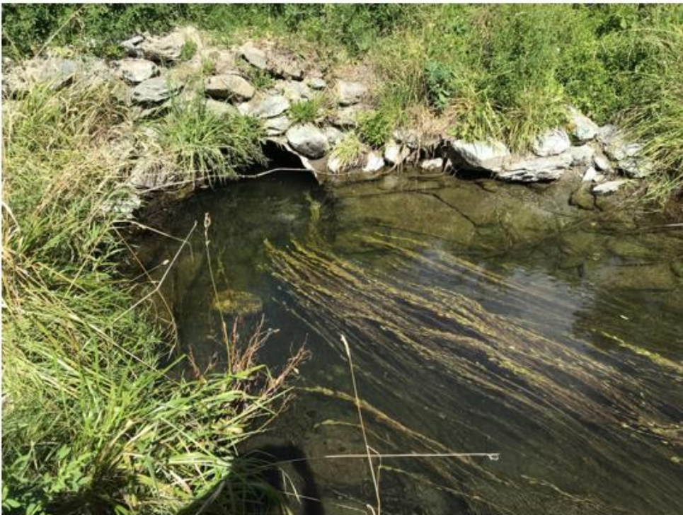
Figure 3. Flow in to the culvert
