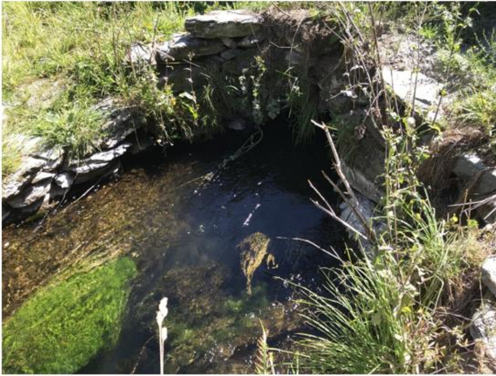
Figure 2. Flow out of culvert
