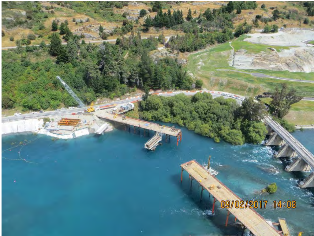
Figure 6: Photograph of temporary platforms - Kawarau Bridge
