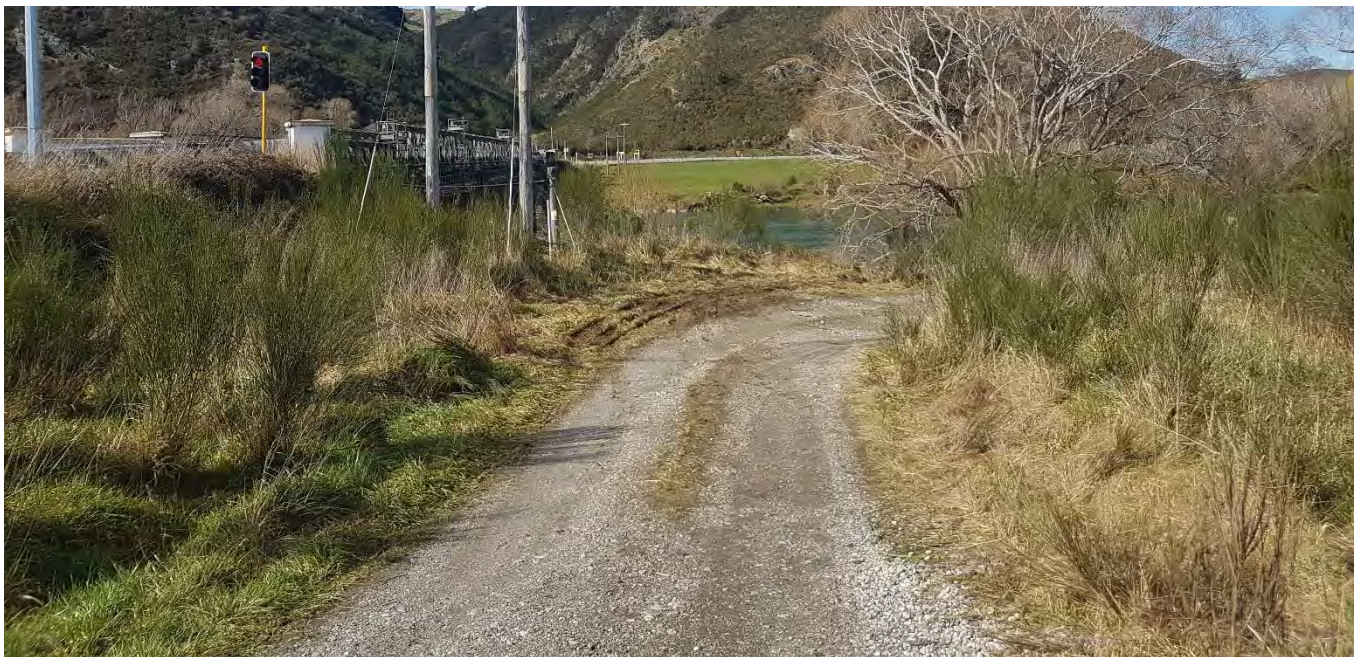
Photo 9: Access road to rest area/ boat ramp
