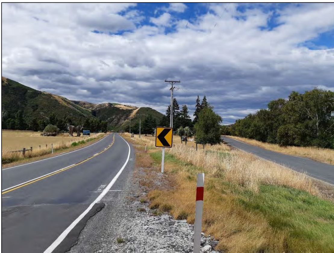
Figure 31. Western extent of the Project area, looking east
