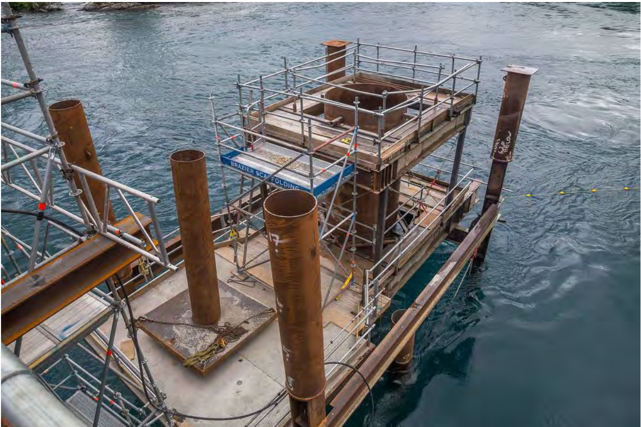
Figure 7: Example of Pile setup
