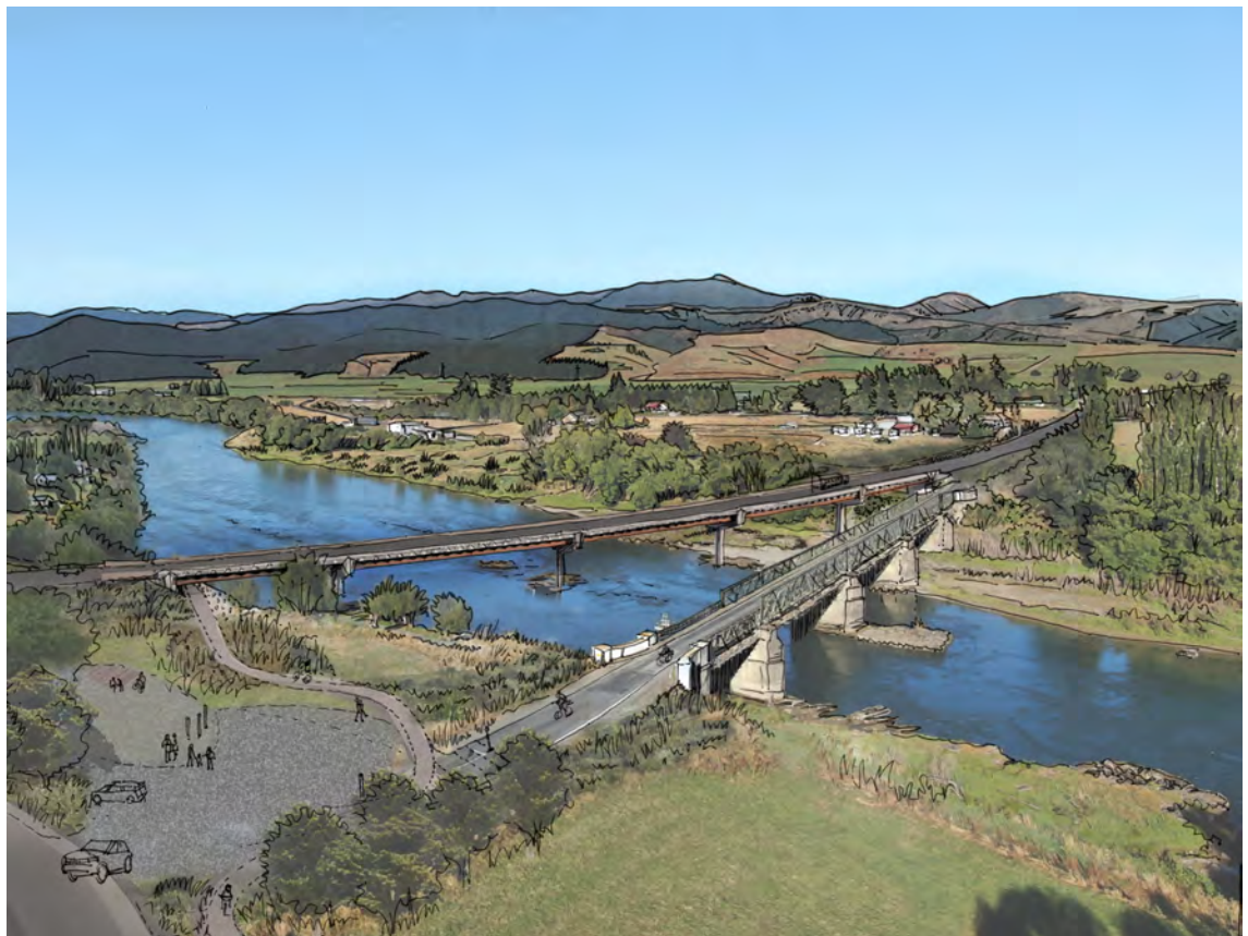
Figure 1 Artists impression of the new State Highway 8 bridge over the Clutha River at Beaumont, looking downstream showing the existing bridge in the foreground.
