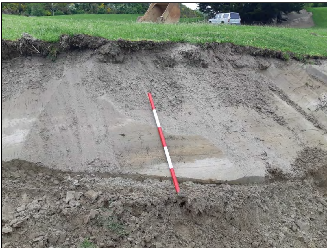
Figure 20. Photograph detailing a batter edge on the true left of the bank of the Mata-au
