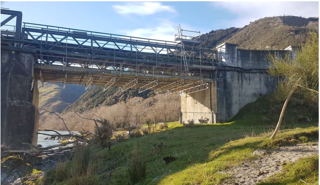
Photo 4: Eastern abutment of existing bridge
