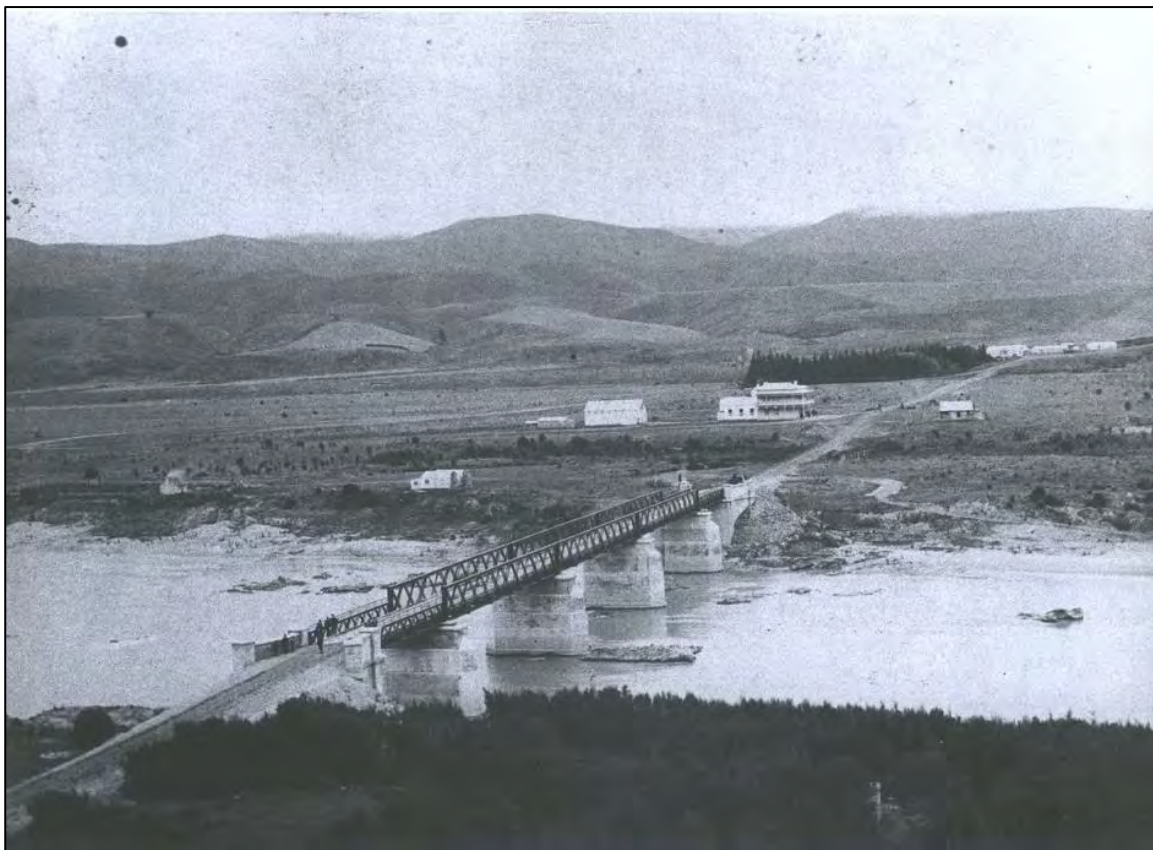
Figure 12. Photograph looking at the second and current Beaumont Bridge c.1890 (source: Hocken Collection Asset ID 6264)
