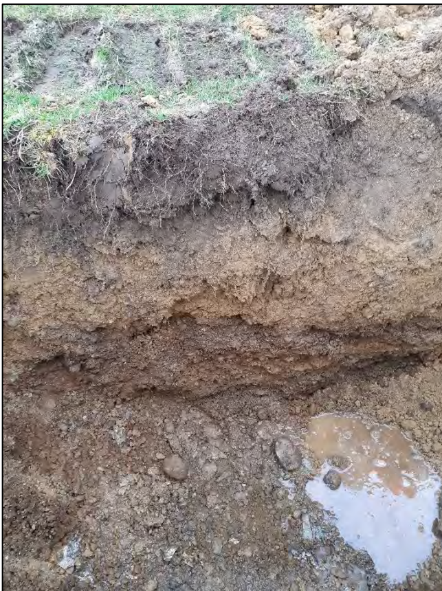
Figure 18. General strata throughout the geotechnical trial pits
